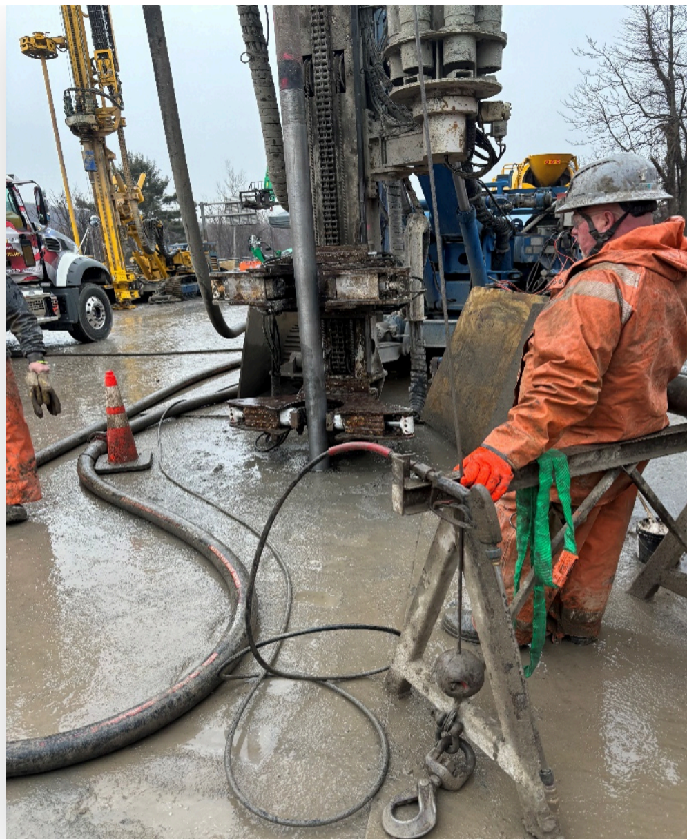
Drilling and Grouting
