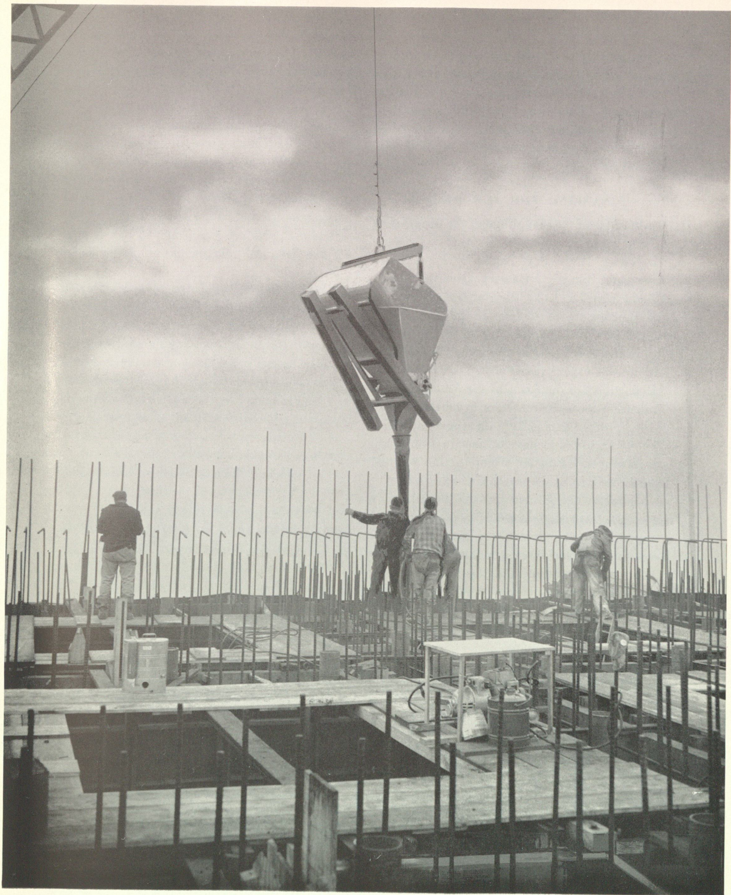
FIRST LIFT OF CONCRETE—GLOUCESTER CAISSON
