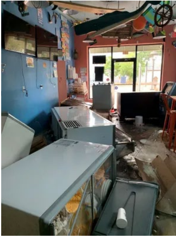
Figure 19: Flood Aftermath at Summer Ville Ice Cream Shop in Somerville, NJ
