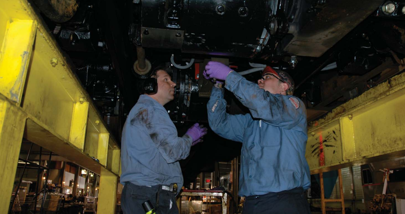
▲ PATCO Motor Repair – PATCO Equipment Mechanics making electrical repairs to a train car.
