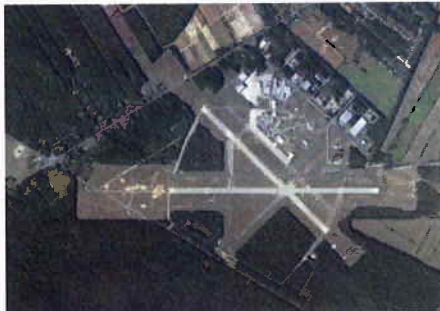
MILLVILLE AIRPORT October 1999
