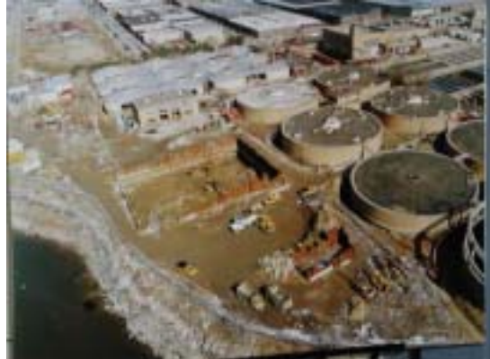
AERIAL VIEW OF ONGOING CONSTRUCTION Photo Courtesy of NYC DEP
