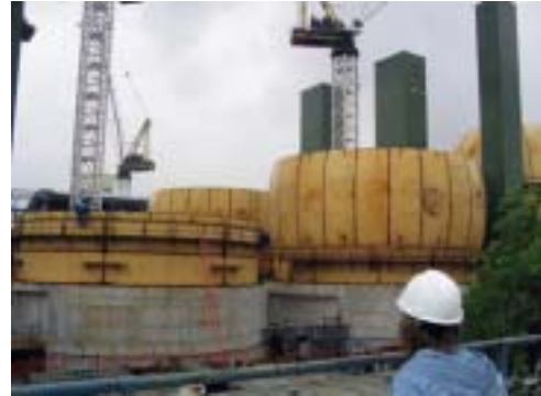
ONGOING UPGRADE CONSTRUCTION
