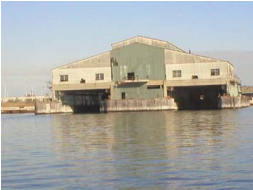
NYC DOS MARINE TRANSFER STATION ON THE EAST RIVER IN THE BRONX, NY
