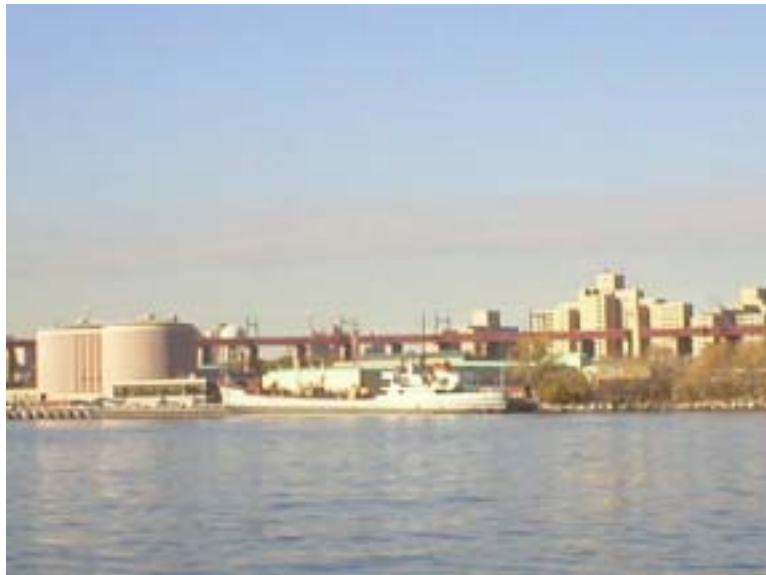
NYC DEP SLUDGE SHIP AT WARDS ISLAND WPCP
