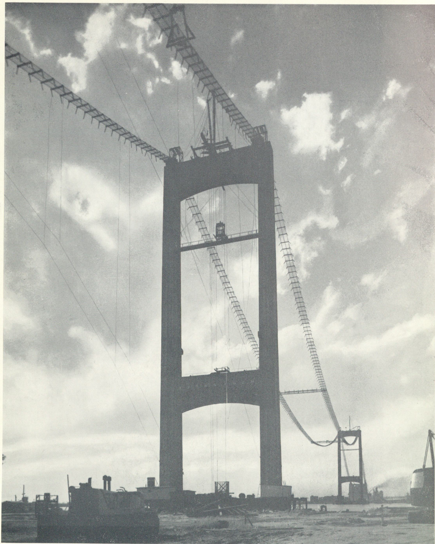
WALT WHITMAN BRIDGE TOWERS AND CABLE FOOTWALKS
