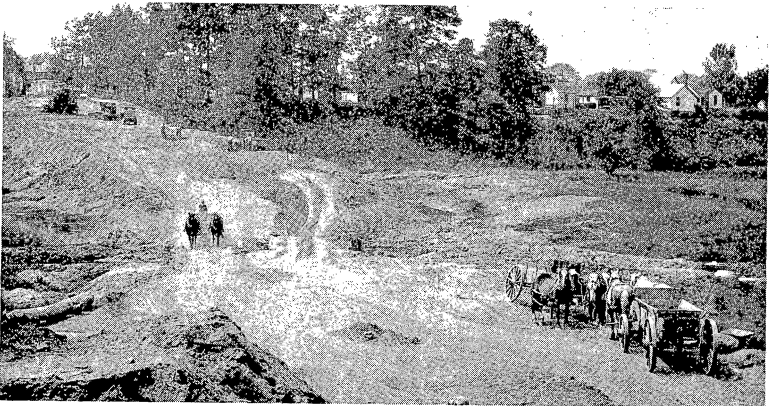
Highway Construction Early 1900s
