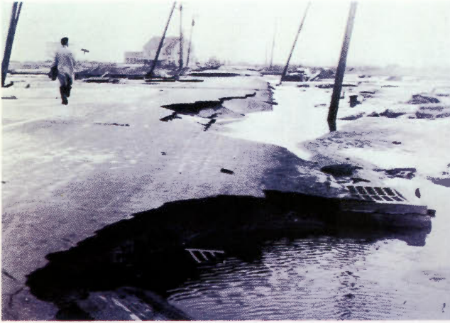
High tides washed out roads and filled them with floodwaters on Long Beach Island
