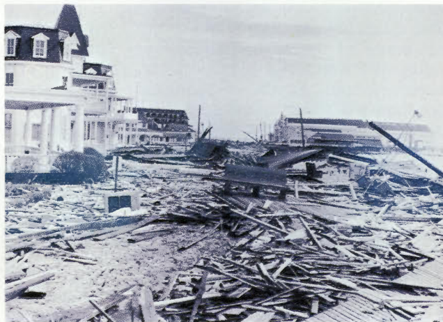
Cape May sustained heavy damages from waves and winds
