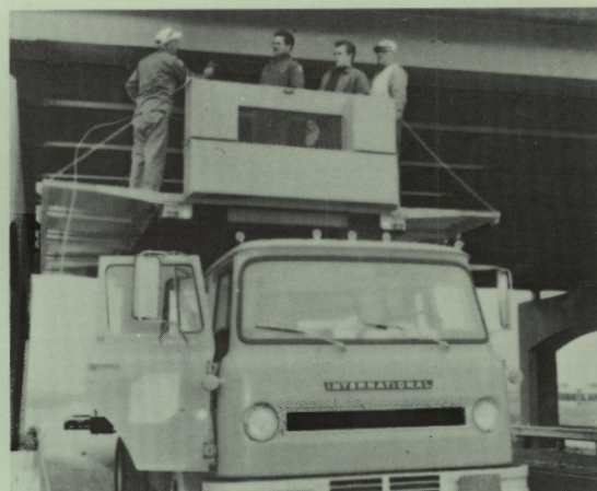
Maintenance crew spray-painting bridge structure at Haddon Twp.
