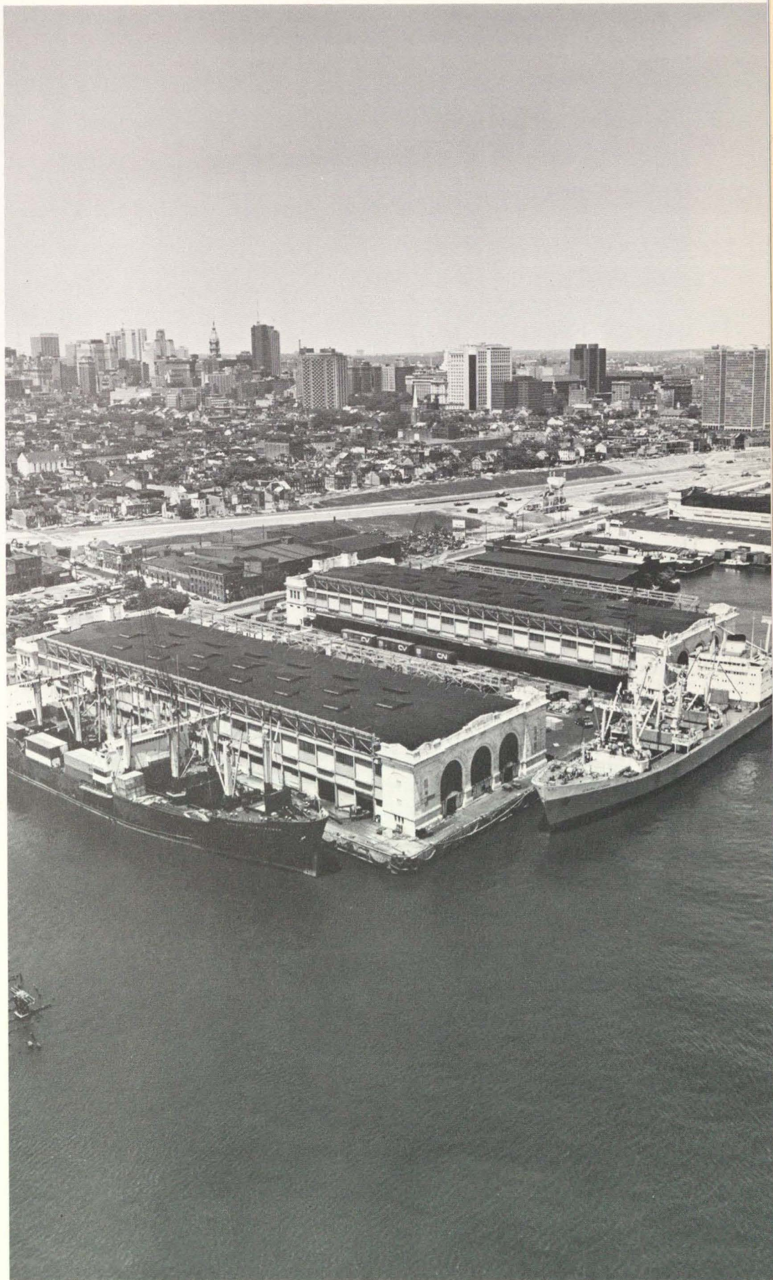
Right: Central Harbor piers adjoin renewal area of Philadelphia with expressway construction in foreground and office buildings at rear.
