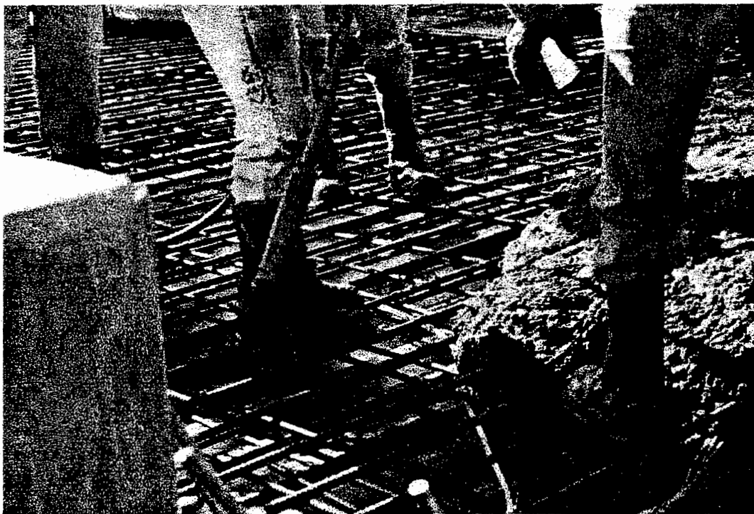
Fig. 3.28: Vibrating of Fresh Concrete at North Main Street Eastbound
