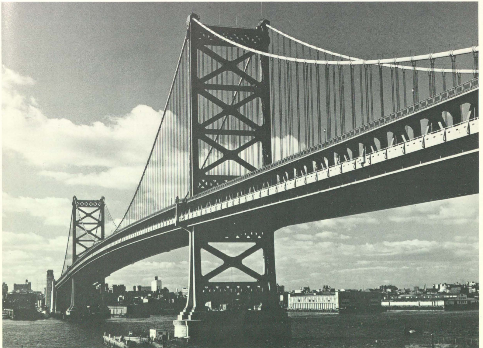
Benjamin Franklin Bridge
