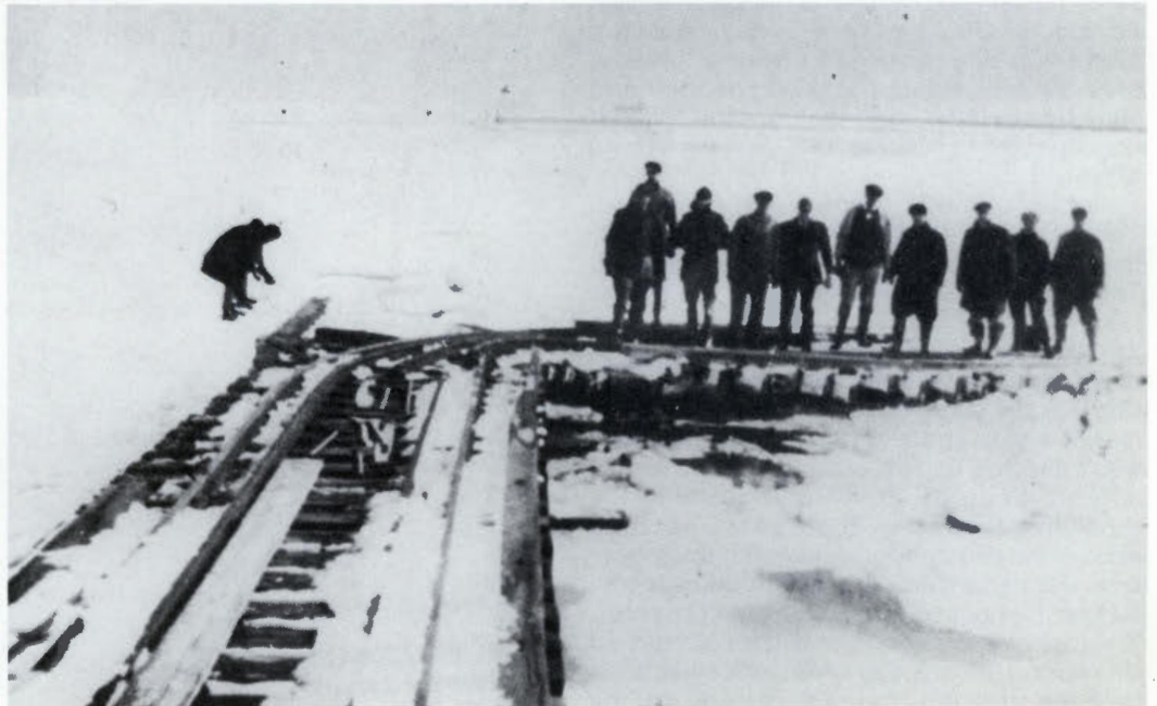
A long trestle over Manahawkin Bay was taken out by ice movement. (circa 1919)
