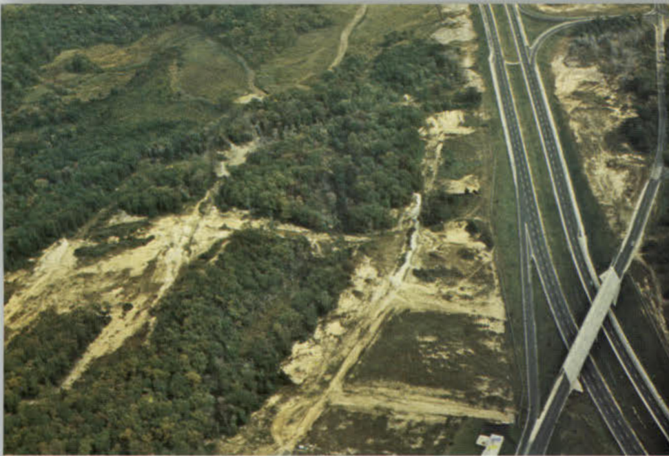
Predevelopment deforestation—drainage from construction site (light area) caused tons of silt to enter a nearby stream (top center).
