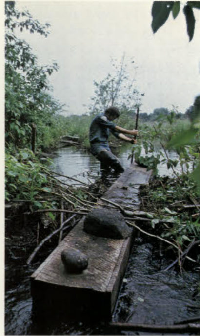
The problem of flooding can frequently be solved with the insertion of a flume in the dam. This keeps the beaver busy damming and maintains the water at a low level.
