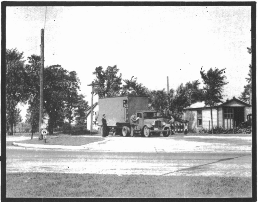
INSPECTORS WEIGHING TRUCKS AND EXAMINING CREDENTIALS AND EQUIPMENT, USING A STATE-OWNED PLATFORM SCALE.
