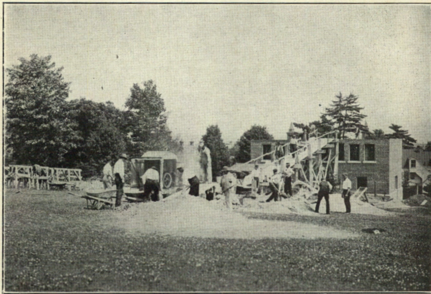
LABORATORY BUILDING FURTHER ADVANCED
