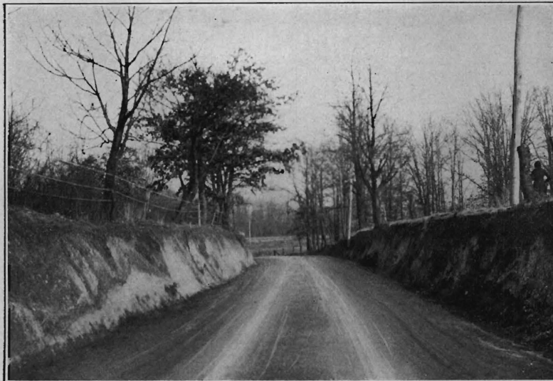
Grover's Mill Road, Mercer County, After Improvement.
