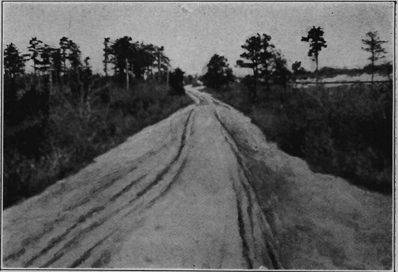
Lacey Township Road, Ocean County, Before Improvement.
