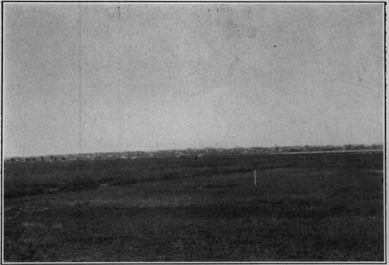
Pleasantville and Atlantic City Boulevard, Showing Meadow over Which Road was Built. Atlantic County.
