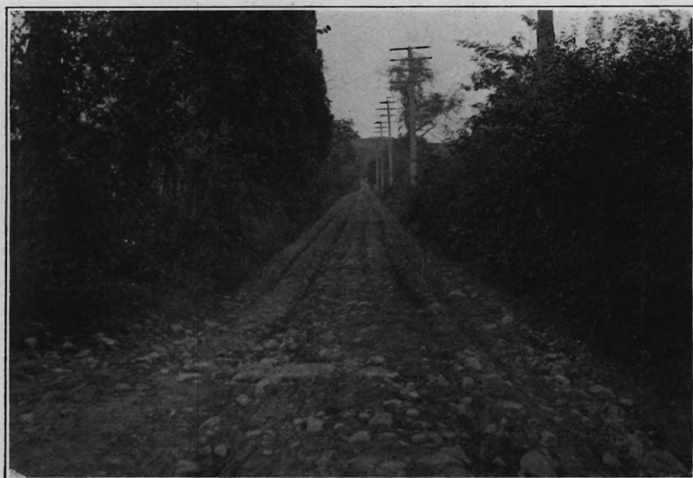
Hobart Gap Road, Essex County, Before Improvement.
