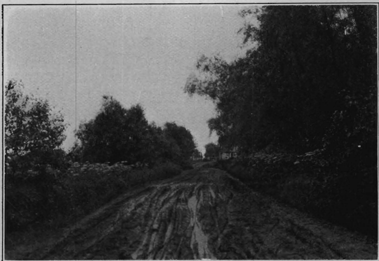
Brunswick Pike Road, Mercer County, Before Improvement.
