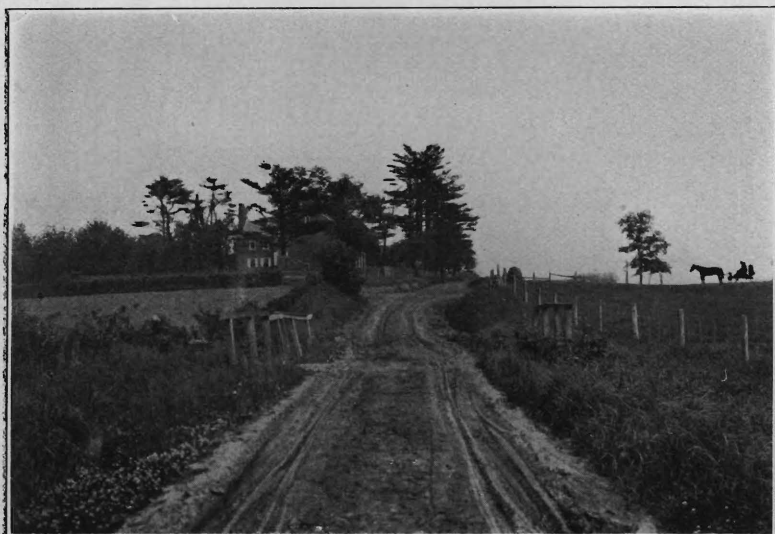
Pennington and Washington's Crossing Road, Mercer County, Before Improvement.
