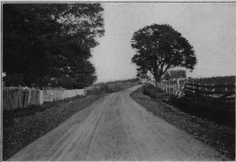
Pennington and Washington's Crossing Road, Mercer County, After Improvement.
