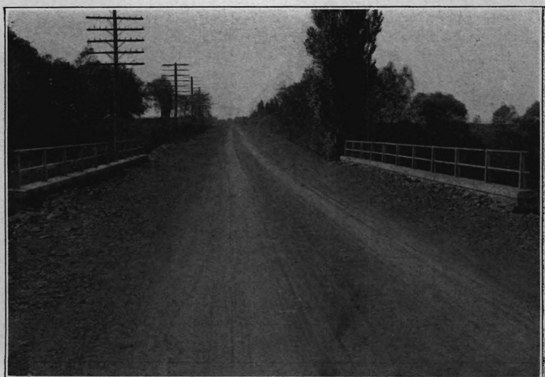
Franklin Park Road, Middlesex and Somerset Counties, After Improvement.
