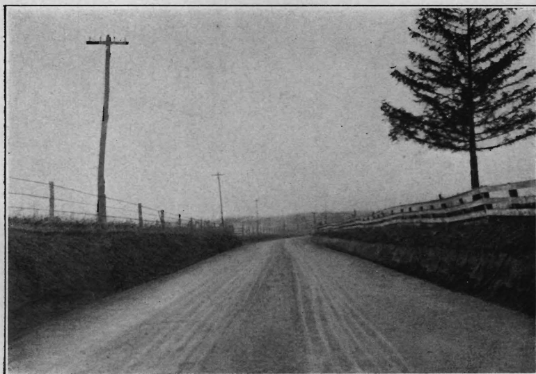
Grover's Mill Road, Mercer County, After Improvement.
