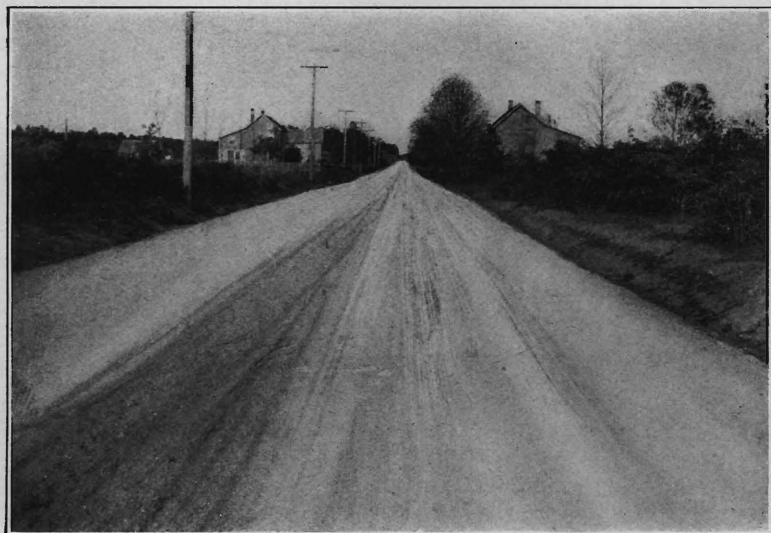
Second Section Stafford Township Road, Ocean County, After Improvement.
