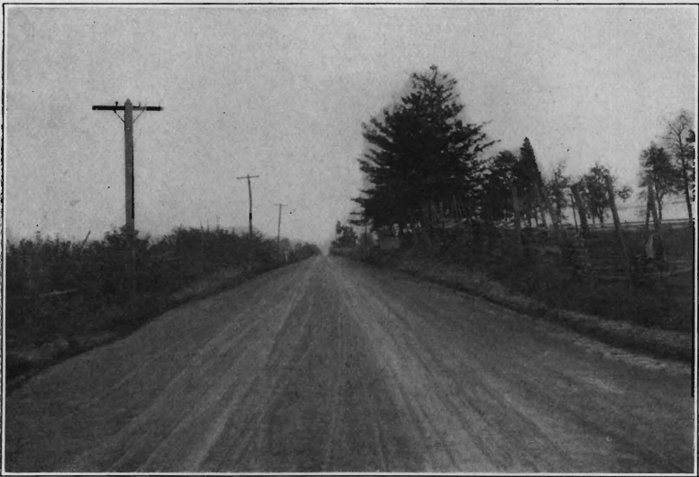
Trenton and Allentown Turnpike, Mercer County, After Improvement.
