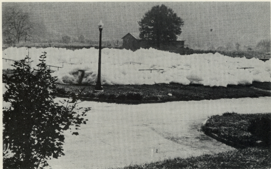
Detergent suds overflowing in a municipal sewage treatment plant
