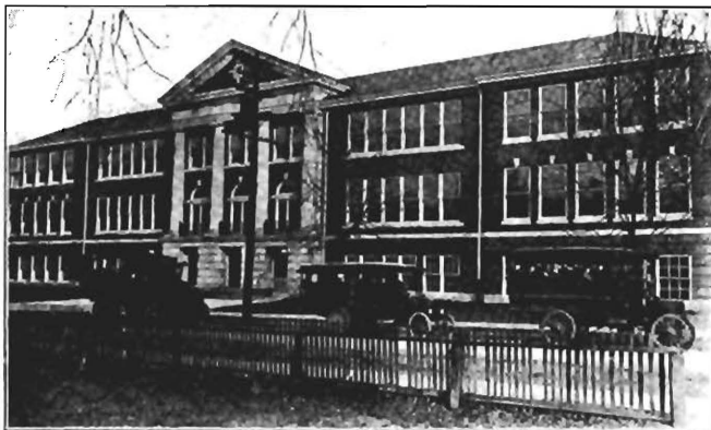
High School 3, Chester Township, Burlington County Contains 16 fine classrooms, large auditorium, offices, manual training room, cooking and sewing rooms. Cost $95,000. Trolleys and three autobusses transport pupils to this school.
