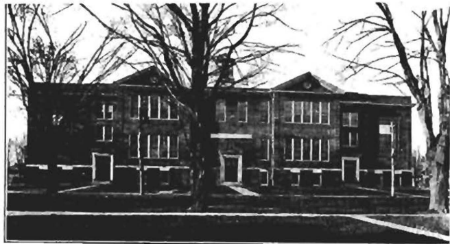
High and Elementary School at Hackettstown, Warren Co. Contains 21 classrooms, offices for Board of Education and Superintendent; assembly hall seating 800. There are rooms for domestic science, manual training, play, special recitations, gymnasium.
