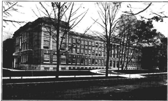
New High School at Montclair Main building contains 72 rooms, including manual training and lunch rooms, teachers', doctors' and study rooms, and laboratories. Auditorium seats 1,200. Cost $560,000.
