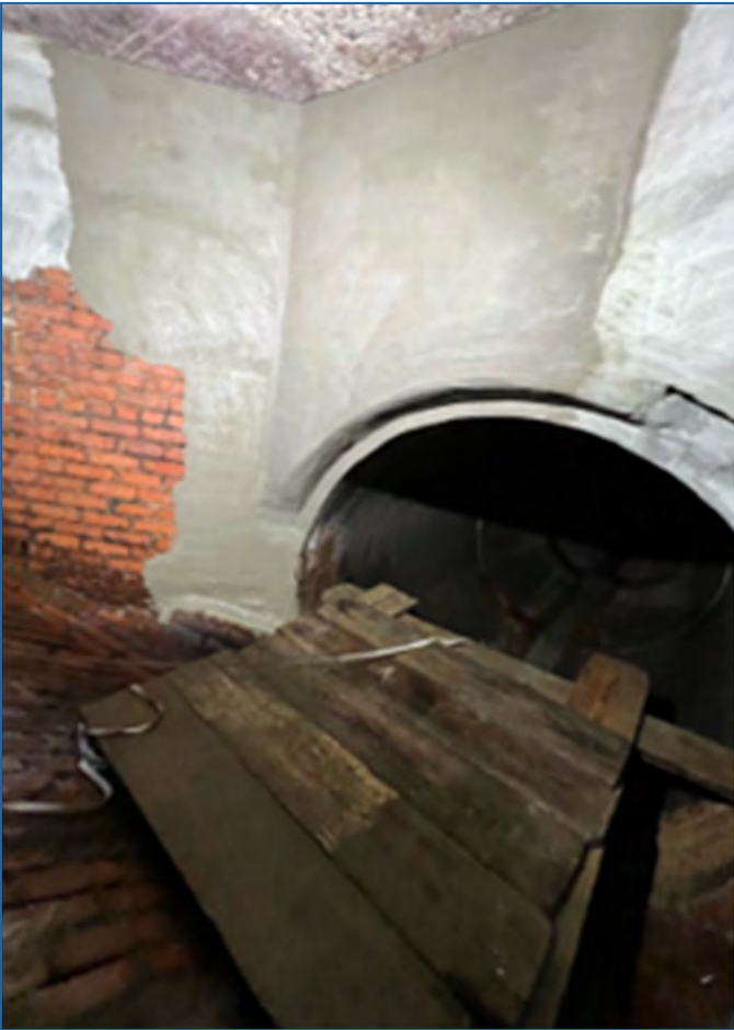
Camden City’s Concrete Restoration
