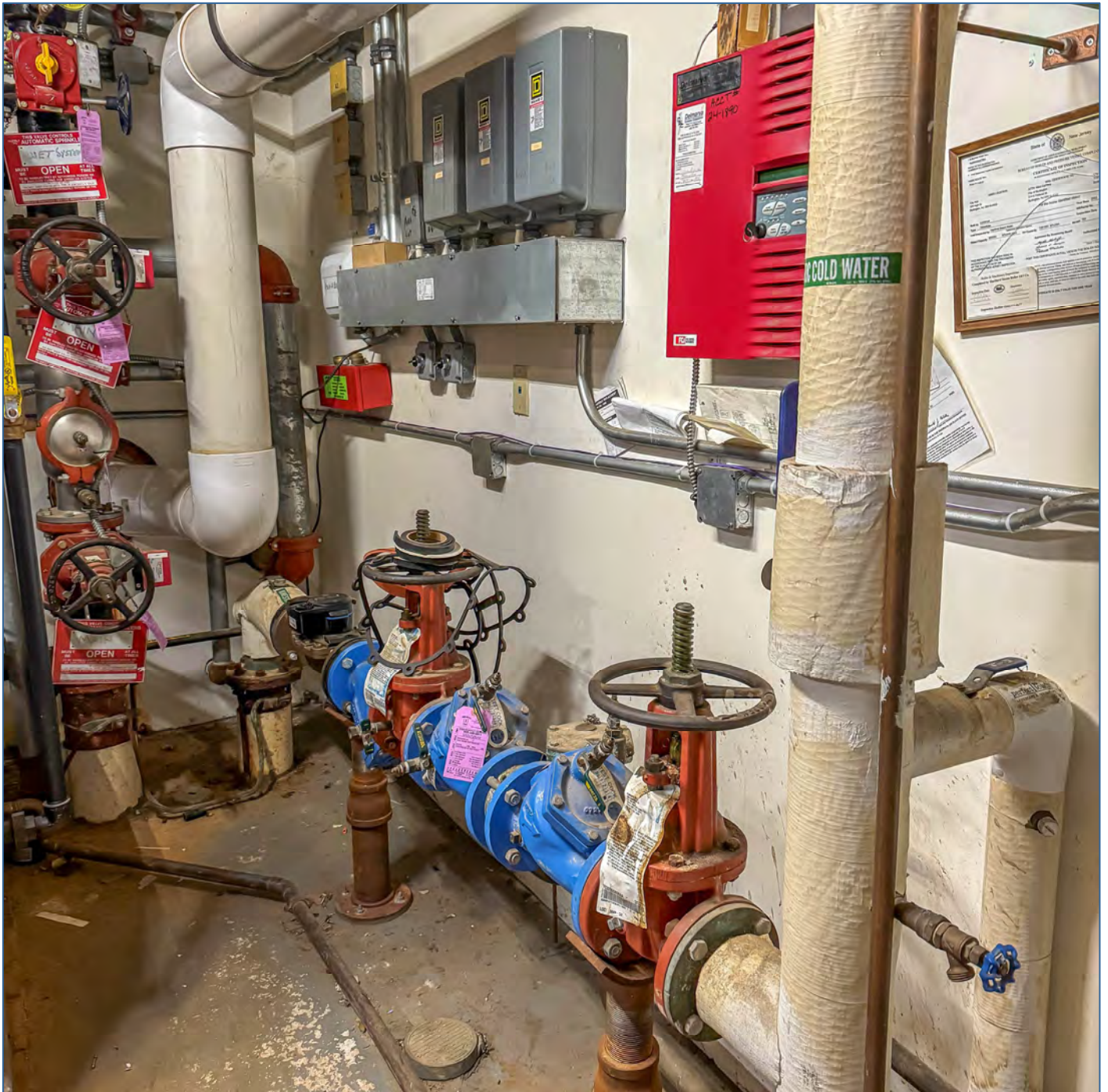
Burlington City: Meter Replacement. SFY2025 Water Bank Long-Term Loan: $1,798,728.
