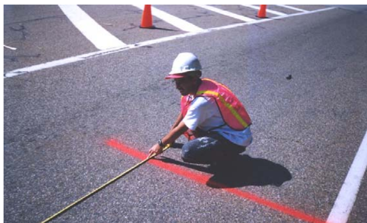
Figure 57 Photograph of the site layout for the installation of the sensors.
