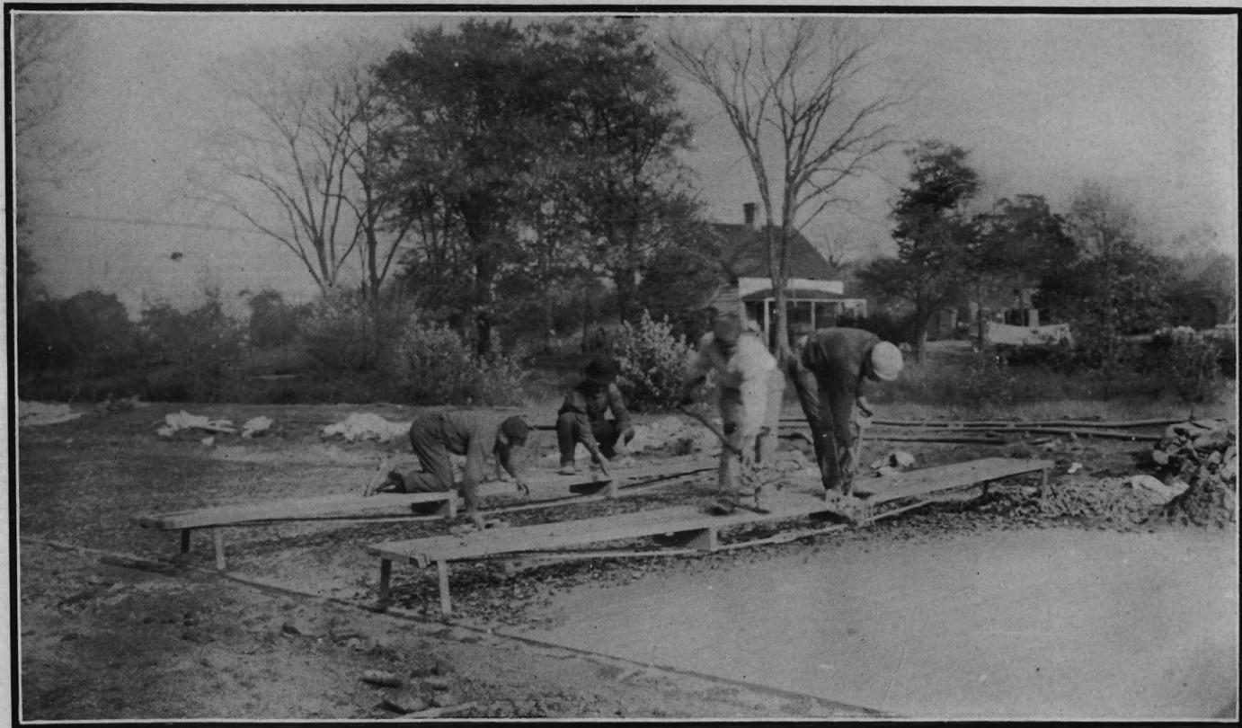
East Broad Street, Westfield, Showing Method of Spreading  $1\frac{1}{2}$  in. Locking Stone on Concrete Base.
