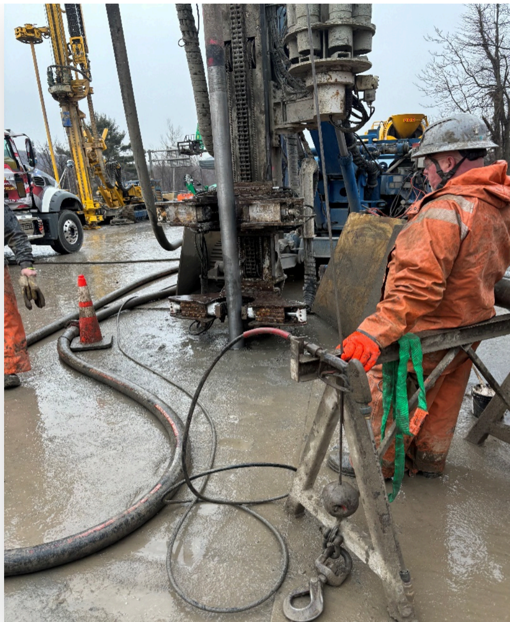
Drilling and Grouting
