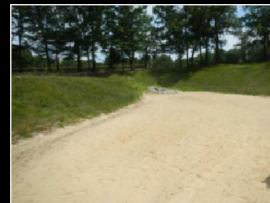
Newly constructed K5 sand lined basins
