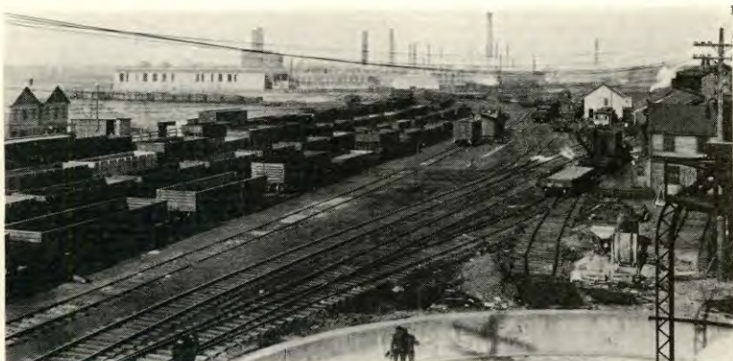
Lehigh Valley Yard, Perth Amboy, to be crossed by bridge.
