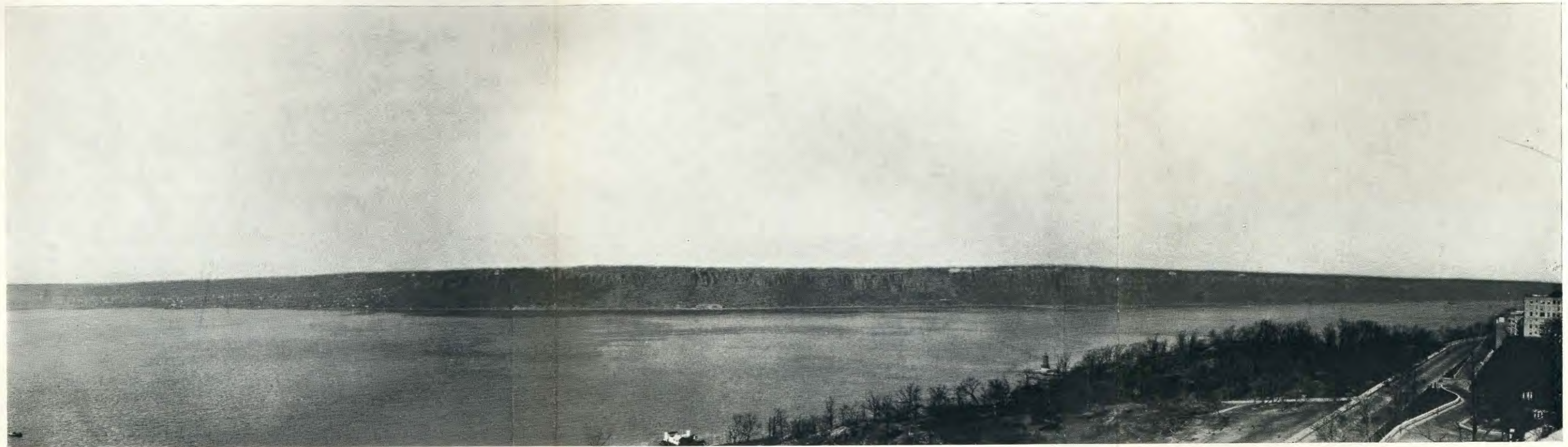
Panorama of the Hudson where the new bridge will cross, looking from Manhattan to New Jersey.
