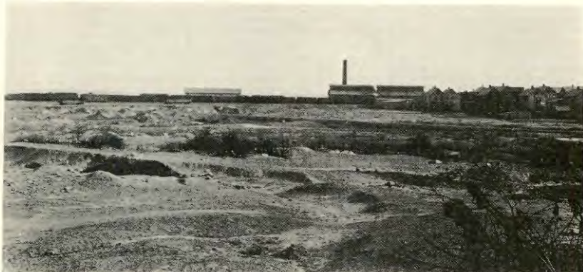
Perth Amboy near center line of bridge to Tottenville.
