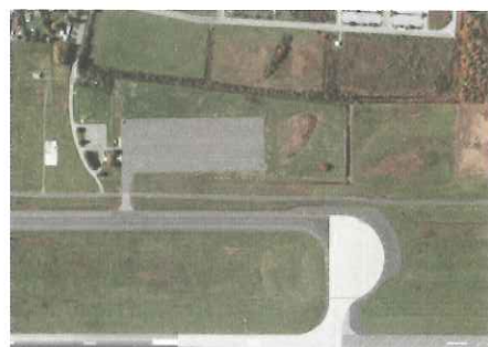
CIVIL AIR TERMINAL August 1999
