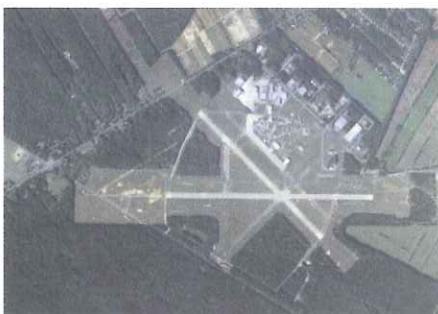
MILLVILLE AIRPORT October 1999
