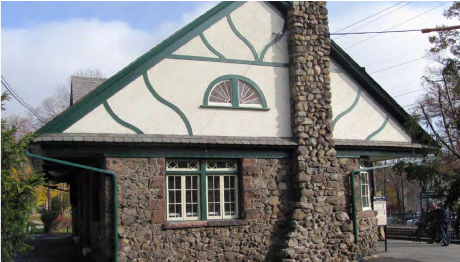
...a state-of-good-repair project led by NJ TRANSIT employees.
