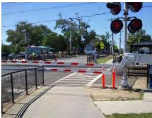
Rail crossing “gate skirts” pilot program
