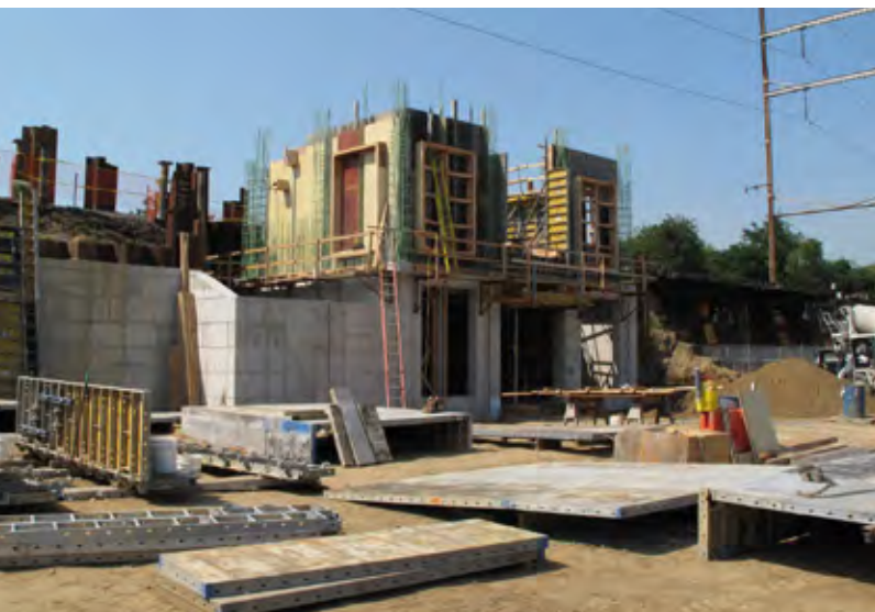
Construction is underway on Pennsauken Transit Center.
