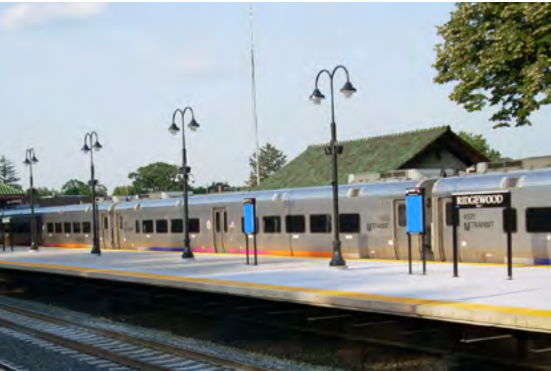
New high-level platforms at Ridgewood Station on the Main Line.
