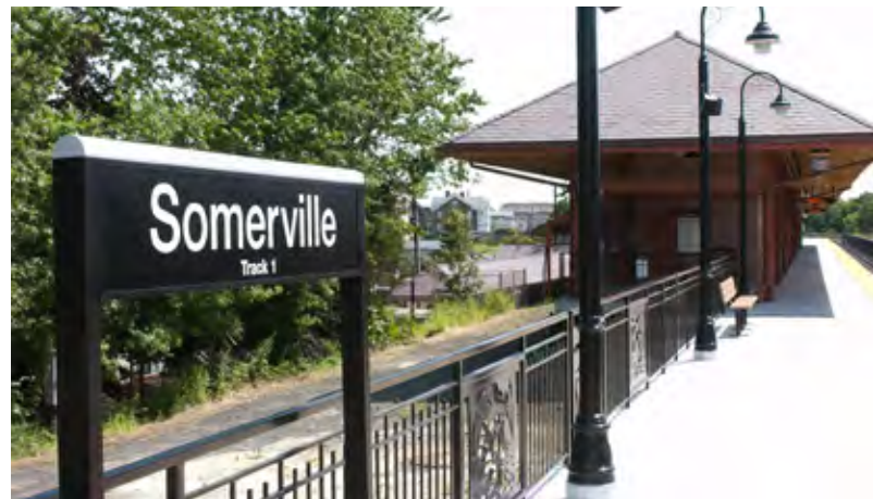
New high-level platforms at Somerville Station were completed on the Raritan Valley Line.
