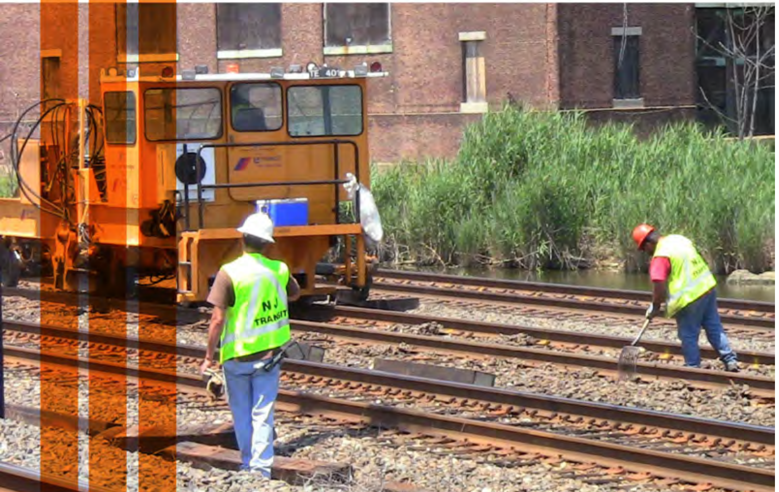
Track maintenance improves service reliability, a key driver for Scorecard .
