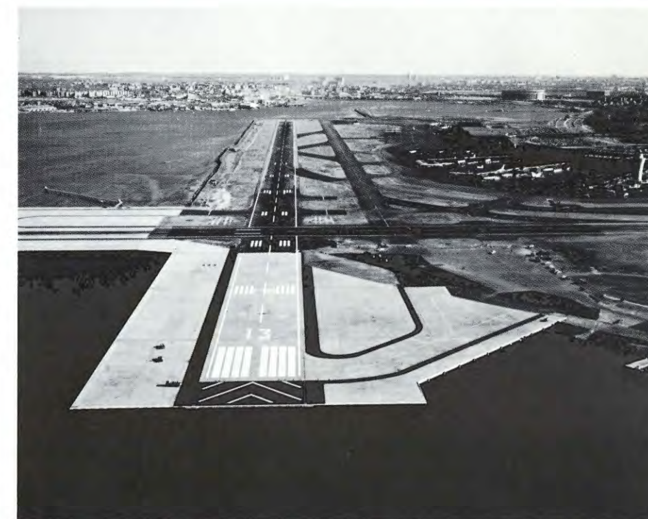
Pilot's eye-view of the recently completed over-water runway extension at LaGuardia Airport.
