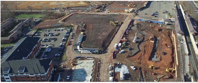
SOMERVILLE STATION BEFORE
