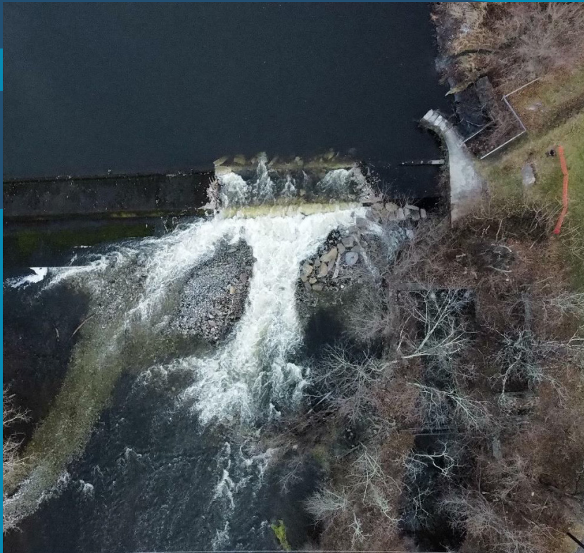
Completed in 2024, the Paulina Dam removal reopened miles of river for fish passage, strengthened watershed health and expanded recreational opportunities along the Paulins Kill. Credit: The Nature Conservancy
