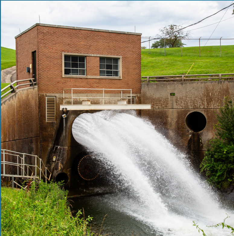
A water release at Spruce Run Reservoir in Clinton. This reservoir is considered one of the first water supply facilities to be constructed and operated by the state.
