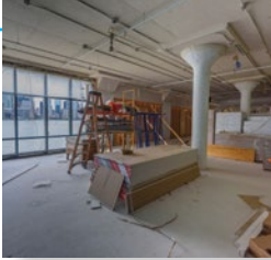
New Jersey City University School of Business construction
