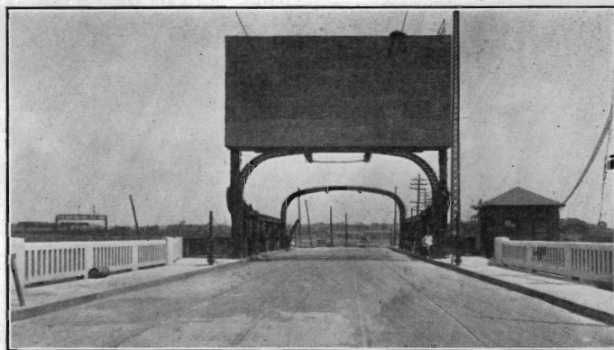
NEW WOODBRIDGE CREEK BRIDGE
