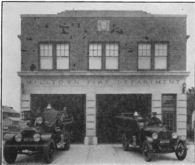
MILLTOWN'S EFFICIENT FIRE DEPARTMENT
