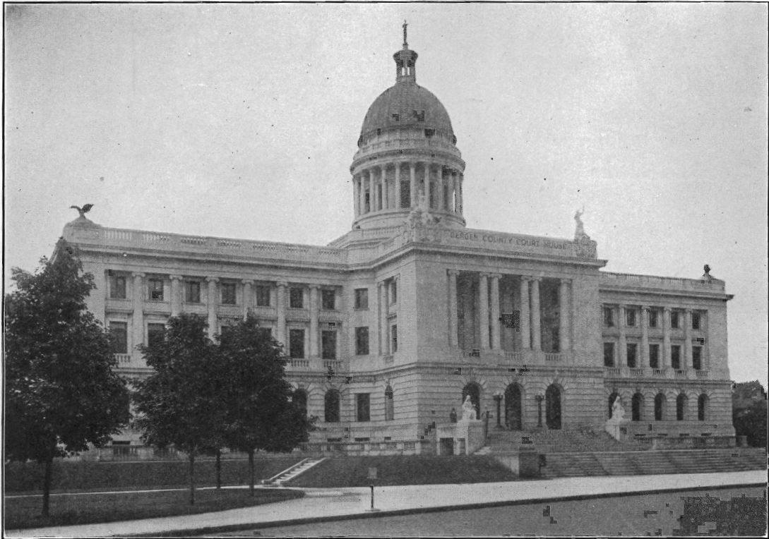
BERGEN COUNTY COURT HOUSE, HACKENSACK, N. J.
