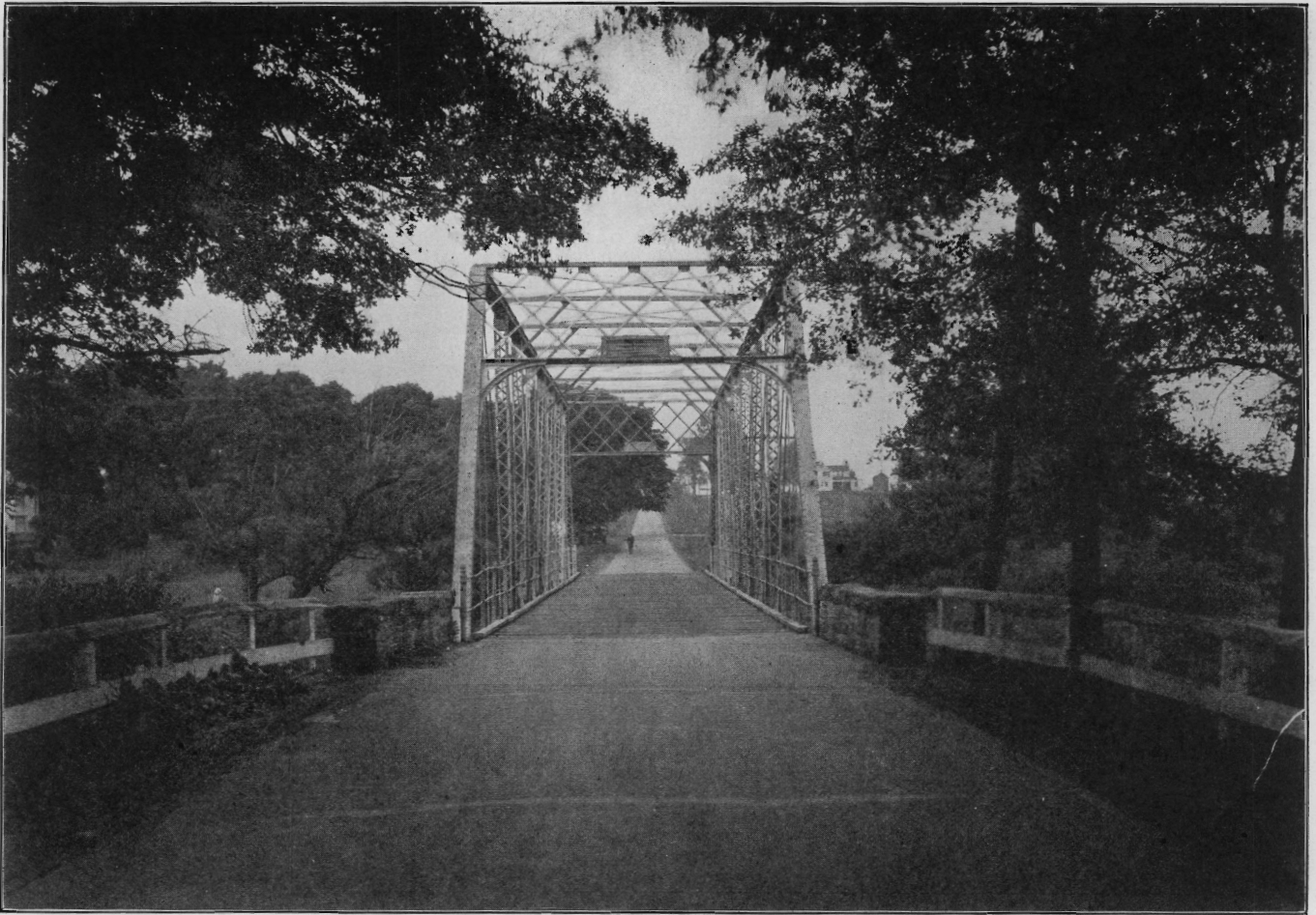
ONE OF MANY WELL KEPT BRIDGES IN MIDDLESEX COUNTY
