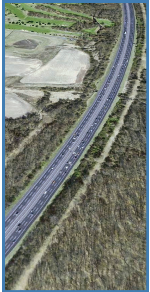
6 LANE ROADWAY - Existing NJ Turnpike South of Interchange 8A prior to proposed widening.
