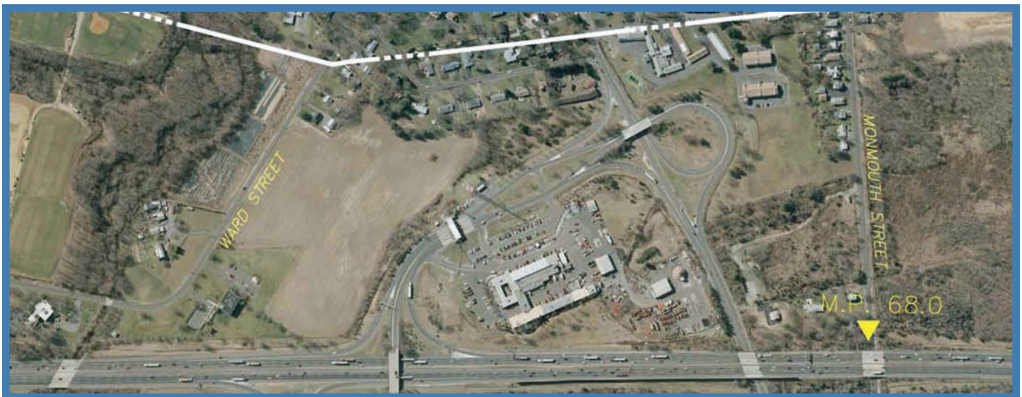
EXISTING INTERCHANGE 8 - The above photograph depicts the layout of Interchange 8 as it now exists prior to final design and construction of the relocated Interchange 8.
