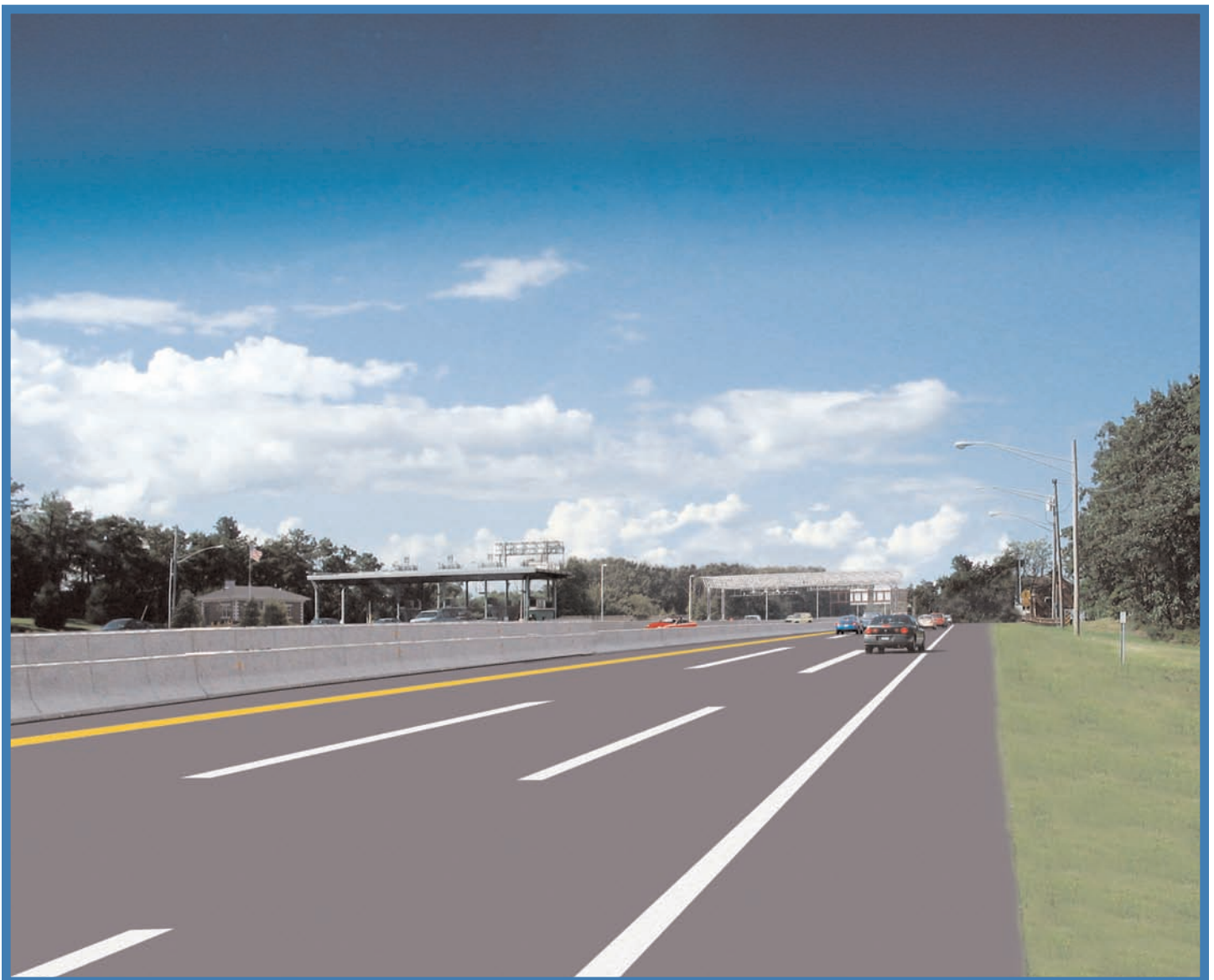
ARTISTS RENDERING - Future condition of Barnegat Toll Plaza. One way tolls, with northbound toll lanes removed and southbound Express E-2Pass lanes provided.
