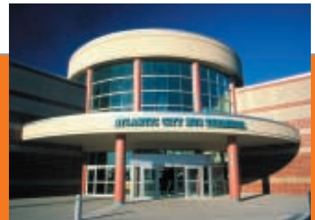
1997 ■ New Atlantic City Bus Terminal opens
