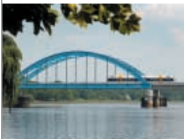
The reconstructed Rancocas Bridge allows rail and marine traffic to operate simultaneously, eliminating delays caused by bridge openings.
