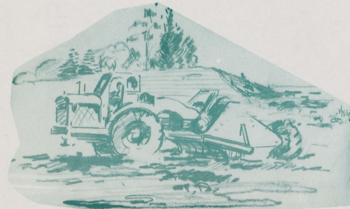
Mountains of earth and rock are moved in rough grading.
