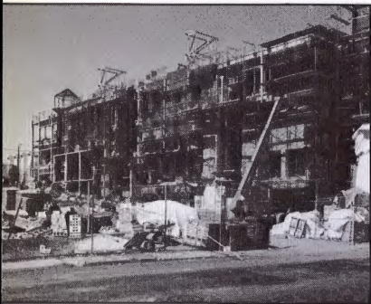
New Jersey Institute of Technology Advanced Technology Center
