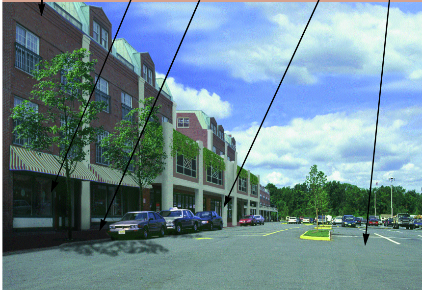
Stage 1 - Redevelopment of Building
