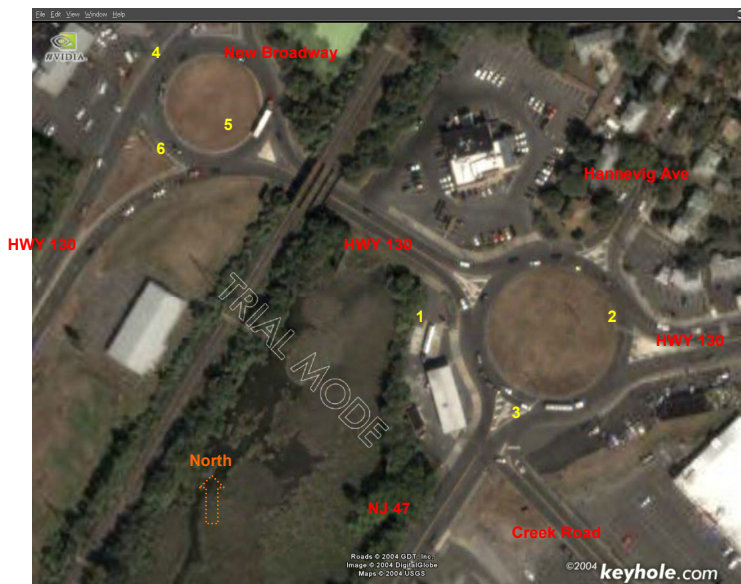
Figure 5. Aerial photo of the Brooklawn Circle
