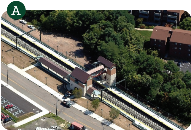
Bay Street Station 23
