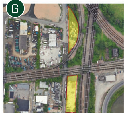
Van Keuren Ave (Jersey City) Semicircular parcel currently serves disorganized truck storage/parking, with potential for 80 parking spaces. It is a southerly parcel site of apparent vacant industrial buildings, with potential for 110 parking spaces. It is a heavily industrial area with significant on-street parking for large trucks.
