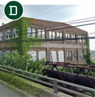
604 Schuyler (Kearny) This building is reminiscent of the park's industrial past and could allow an interior elevator to the park below.
