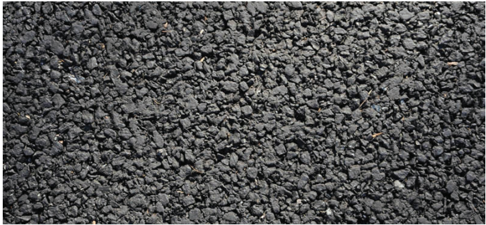
Shared use paths are made with porous asphalt.
