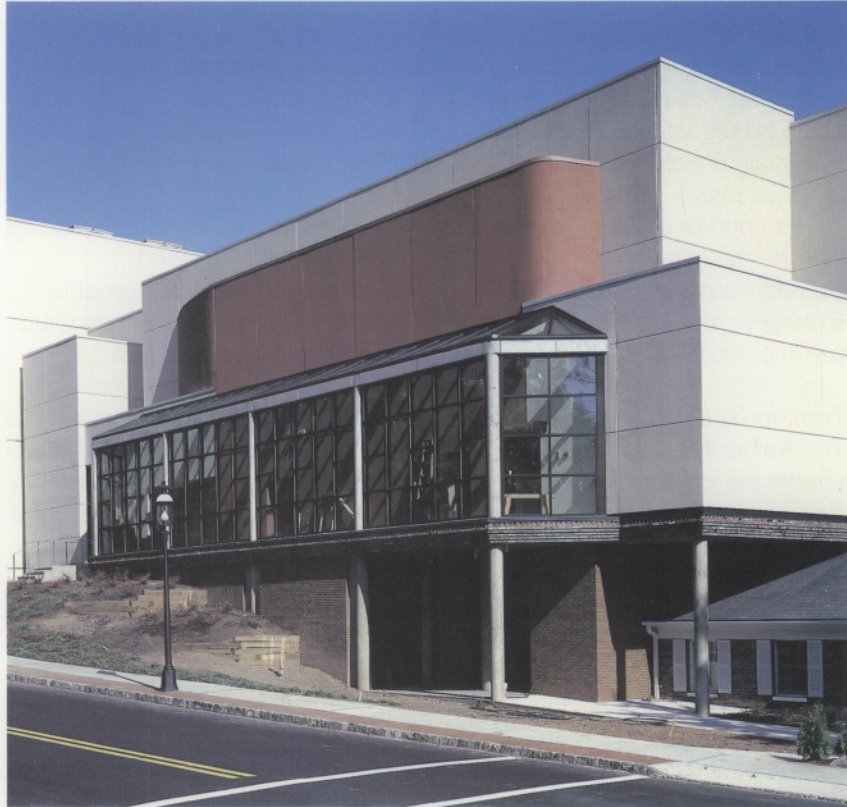
Paper Mill Playhouse, in Millburn, received $2.2 million in tax-exempt financing to rebuild the fire-damaged playhouse.
