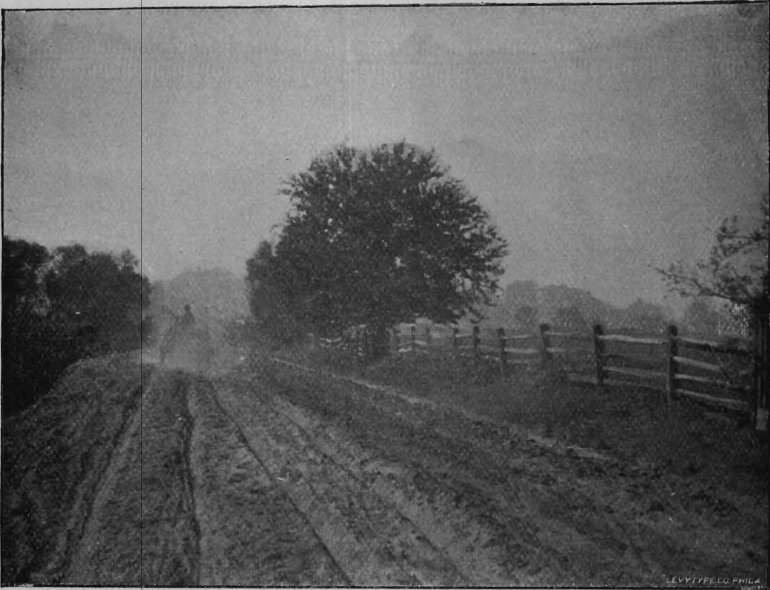
Browning Road, Camden Co. Before.
