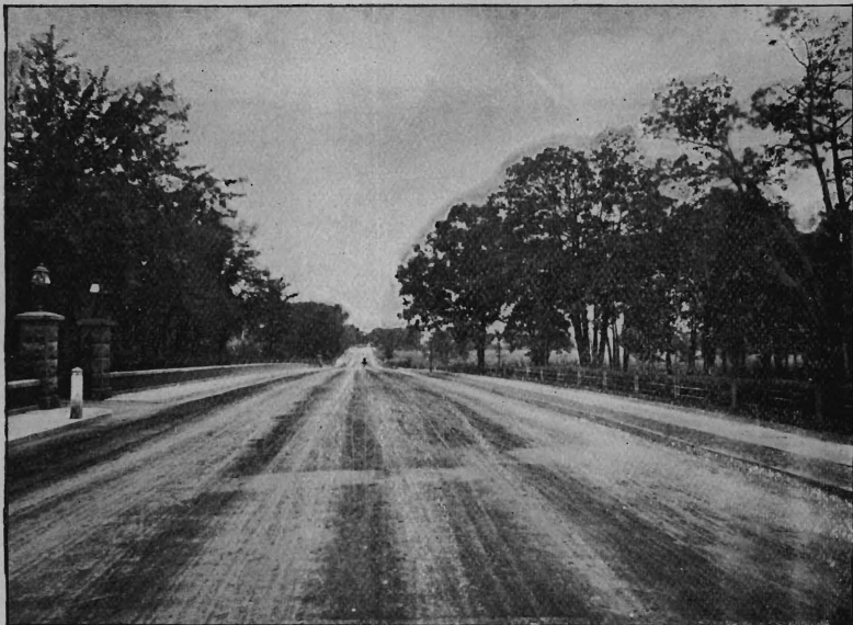
Long Branch and Asbury Park Road, Monmouth Co. After Improvement.
