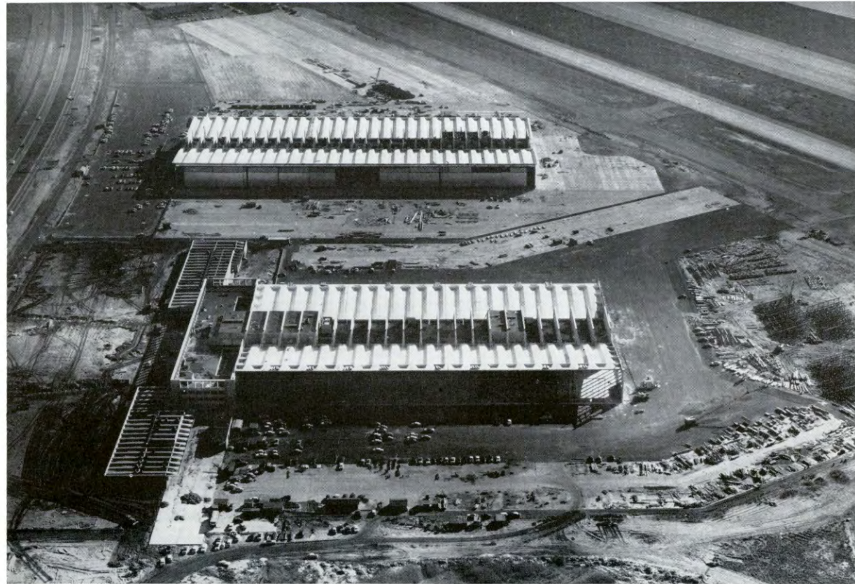
Pan American World Airways Hangar 14 (foreground) and Trans World Airways Hangar 12, have cantilevered concrete roofs over the hangar section. The roofs of these hangars are suspended by tensioned steel cables extending from the center section.
