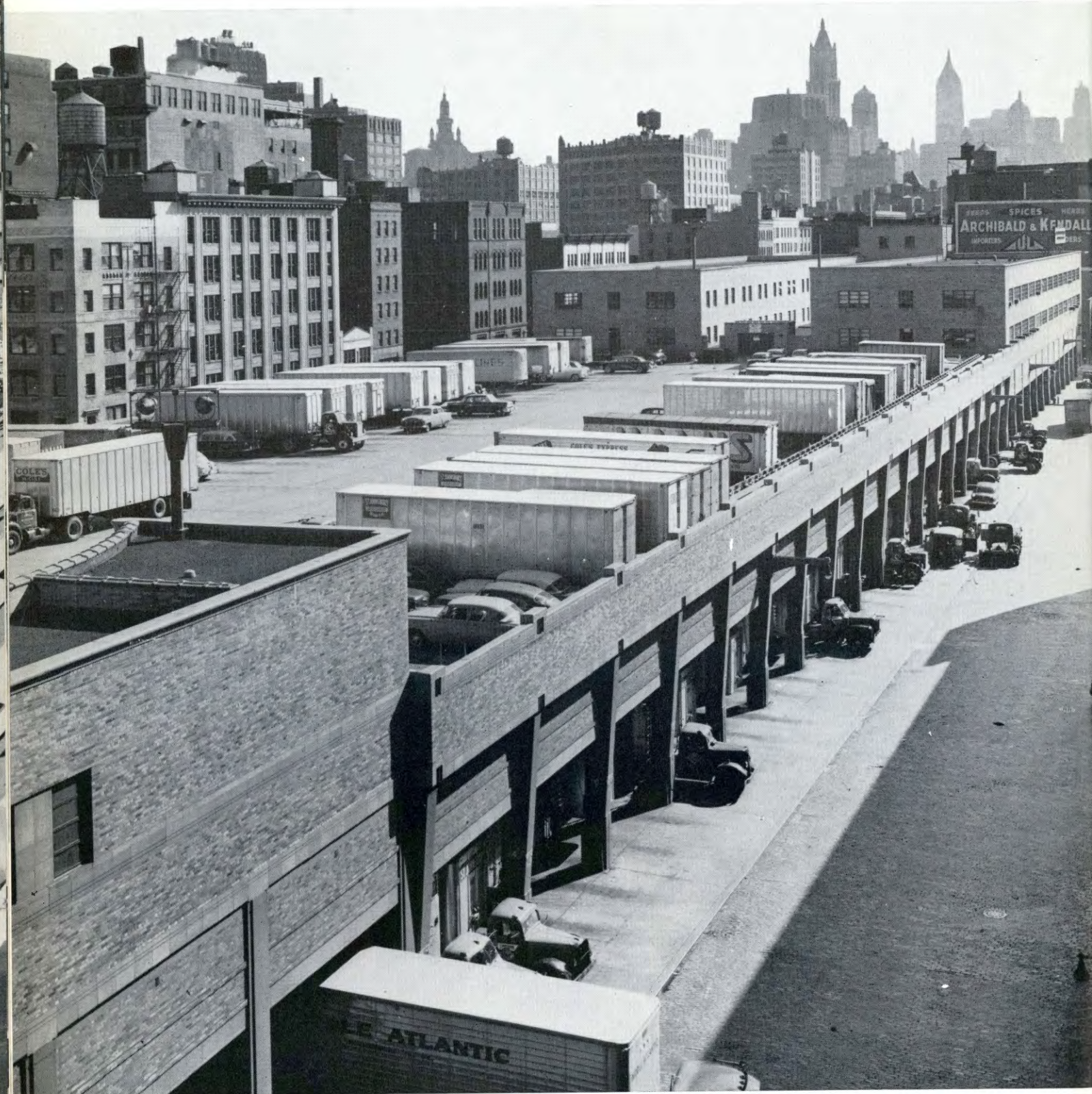
The New York Truck Terminal, conveniently located near the Holland Tunnel, is a consolidated freight receiving and shipping station. Its streamlined operations eliminate pick-up and delivery duplications for the eight carriers of the tenant Empire State Truck Terminal Corporation. It has accommodations for 142 tractor-trailers at one time as well as roof parking for 115 units.
