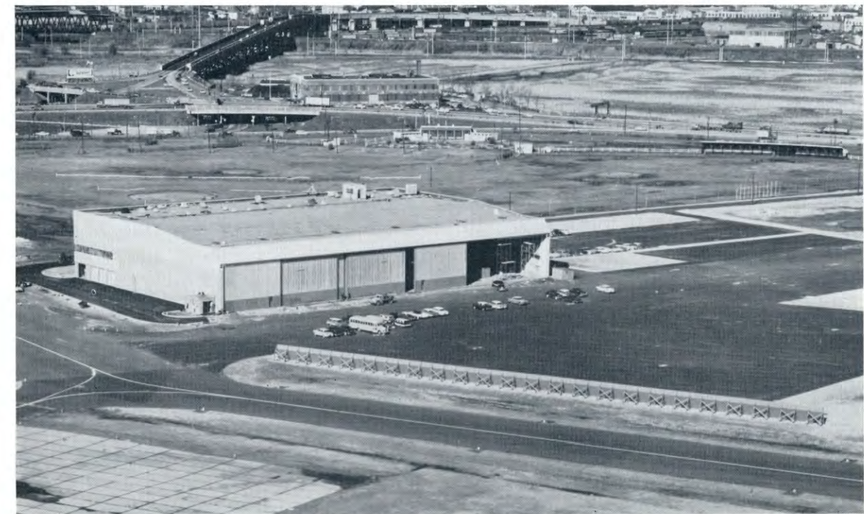
The first major hangar project at Newark Airport in recent years, United Air Line's two-bay cantilevered hangar (left) neared completion during 1957. The $3,750,000 structure and adjacent paved areas are expected to be put into operation by March, 1958.
