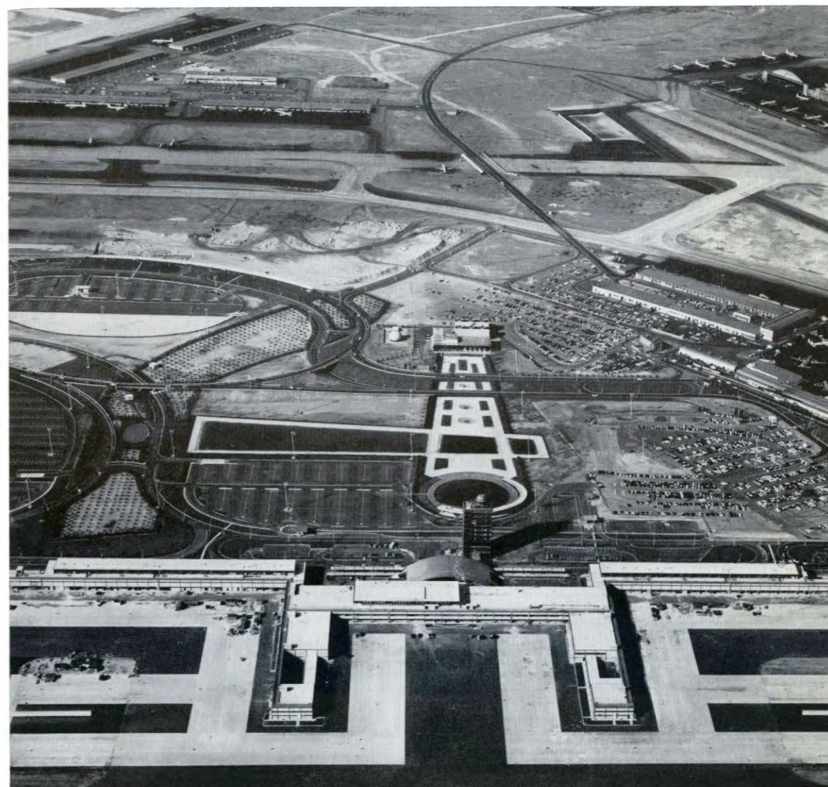
Work on the eleven-block-long $30,000,000 International Arrival and foreign-flag airline Terminal Buildings (foreground), heart of New York International's Terminal City development, was completed in 1957. During construction of buildings, roadways, parking lots and landscaping, traffic at the airport reached a high of 5,193,000 passengers and 206,054,000 pounds of air cargo and air mail.
