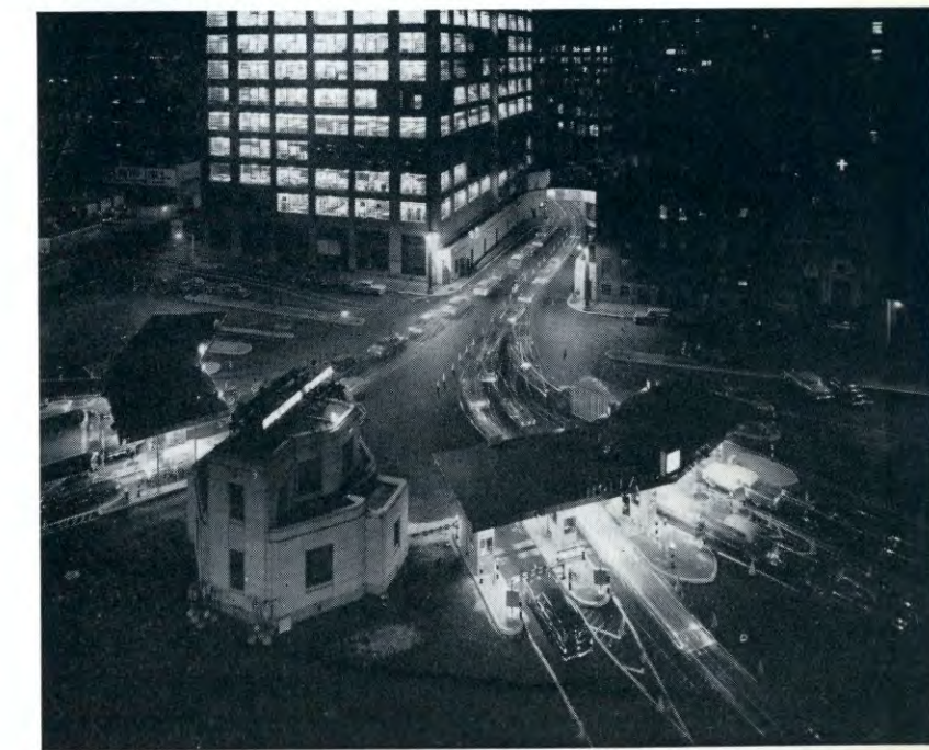
New York Plaza of the Holland Tunnel was modernized in 1957 at cost of $196,000, with installation of eight new toll booths with protective canopies and mercury vapor lighting.
