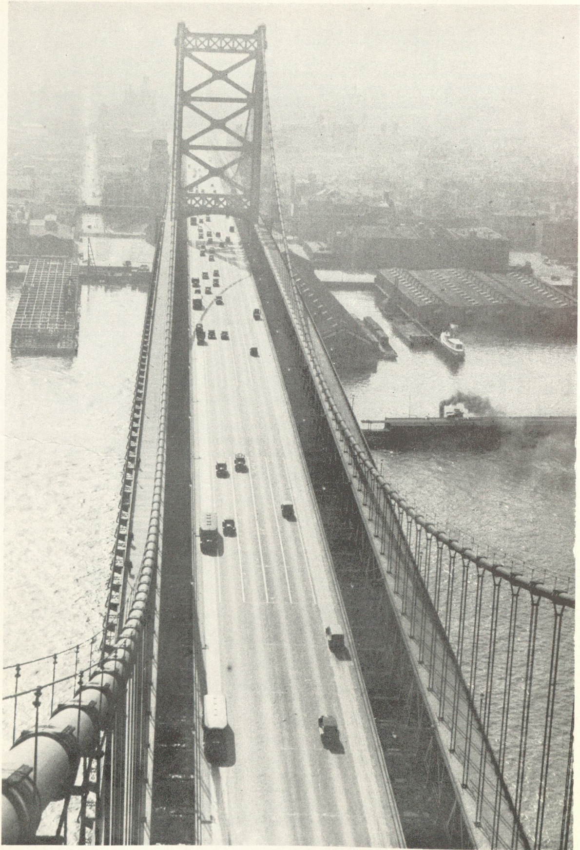
DELAWARE RIVER BRIDGE BY DAY
