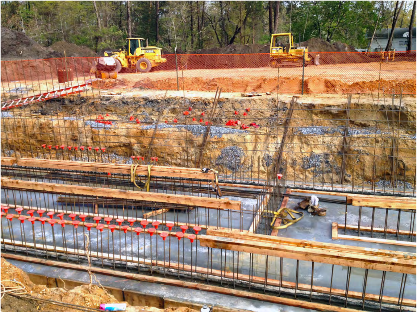
Millville City | Geissinger Well No. 18 Concrete Clearwell Pit Foundation SFY2013 Loan: $2,885,775
