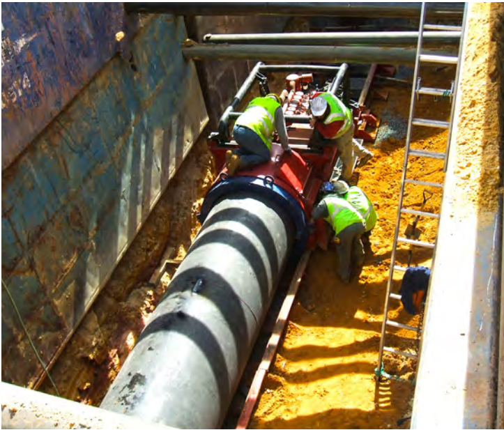
Above: Jack and bore installation of pipeline
