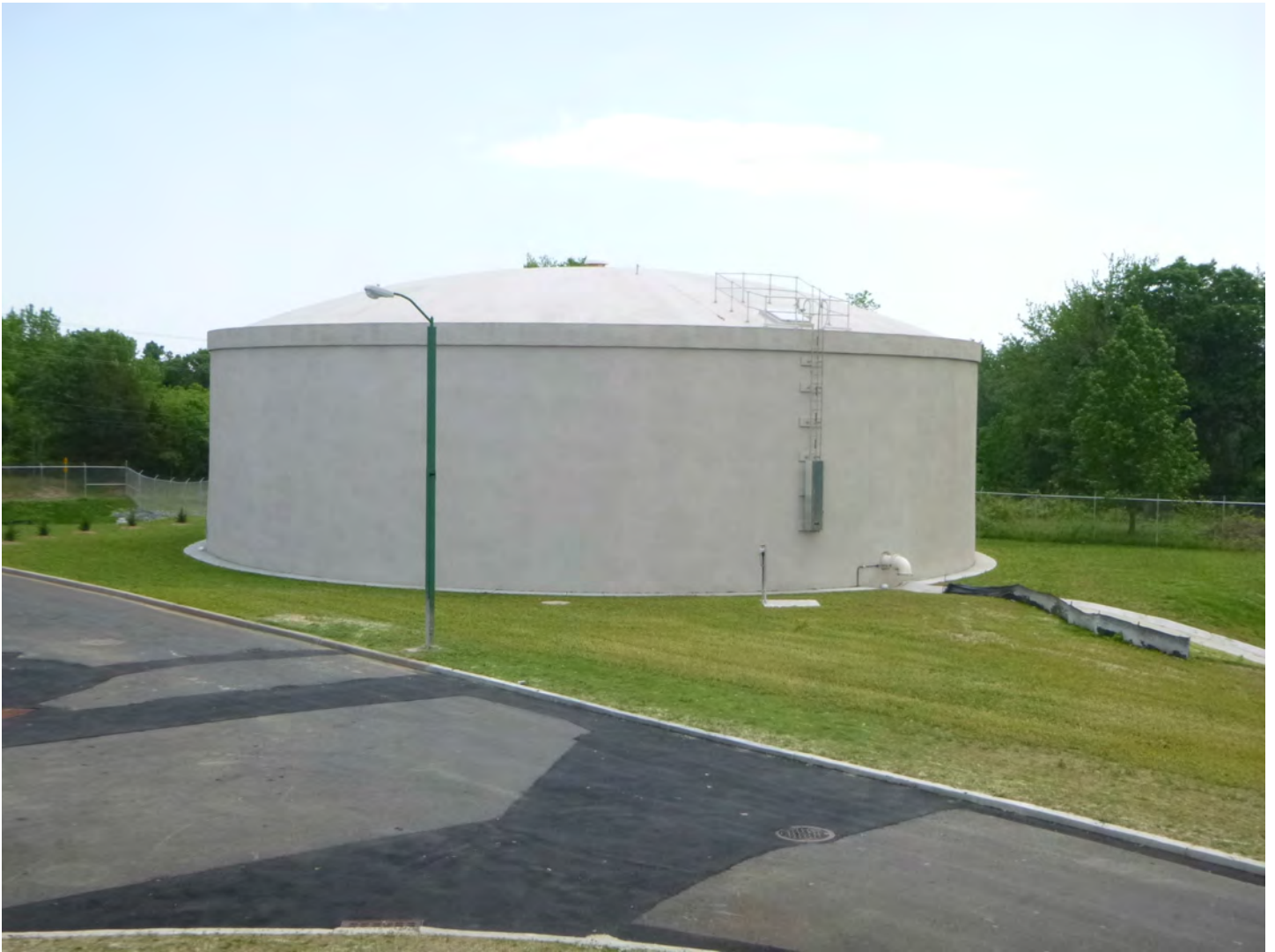
Southeast Monmouth MUA | Manasquan Water Treatment Plant 2M Gallon Ground Level Storage Tank SFY2013 Loan: $8,821,000
