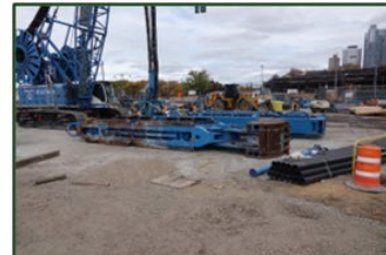
October 29, 2025 Mobilizing slurry wall equipment (Looking Northwest)
