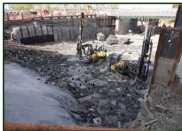
October 28, 2025 Drilling of blast holes (Looking West)
