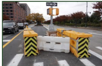
October 29, 2025 Median demo and paving complete (looking South)
