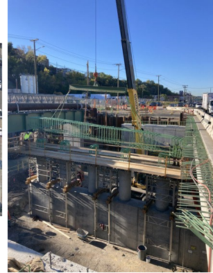
October 17, 2025 Stage 3 – Reinforcement
