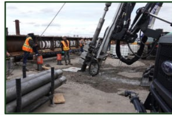
October 29, 2025 Installation of freeze pipe/grout sleeves (Looking West)
