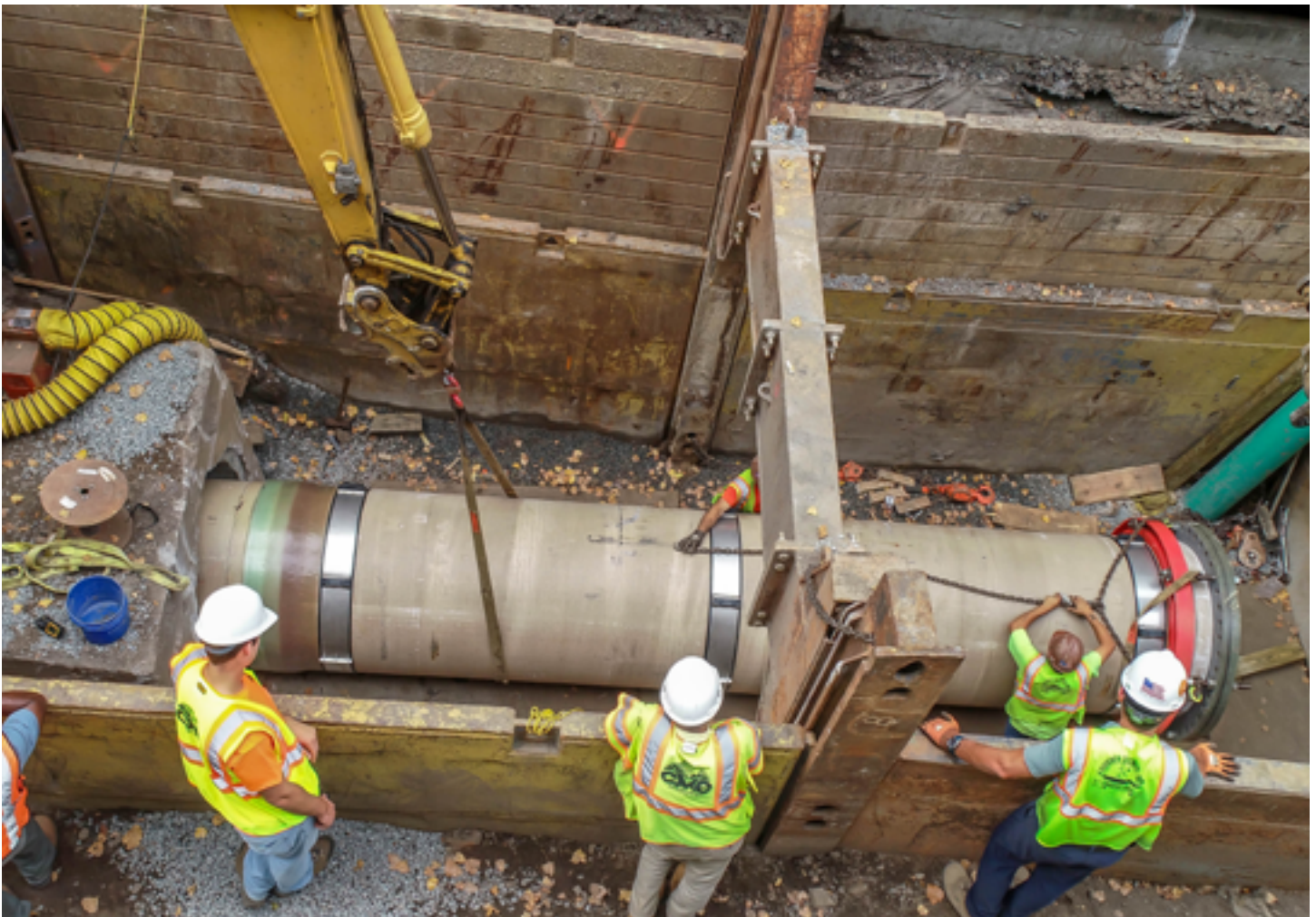
Jersey City MUA, Phase 3 and 4 Sewer Improvements. SFY2021 Loan: $35,669,487
