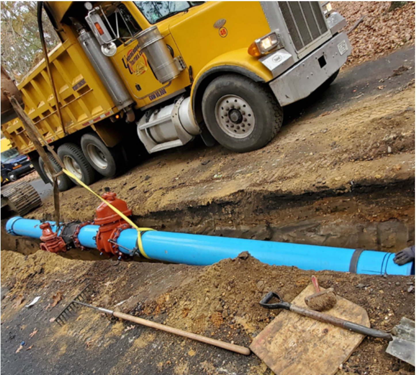
Wall Township, Route 138 Water Main Improvements. SFY2021 Loan: $3,008,598
