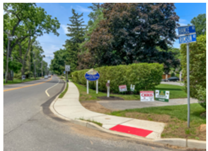
Little Silver, Branch Avenue Sidewalks, Phase II. SFY2021 Loan: $459,000
