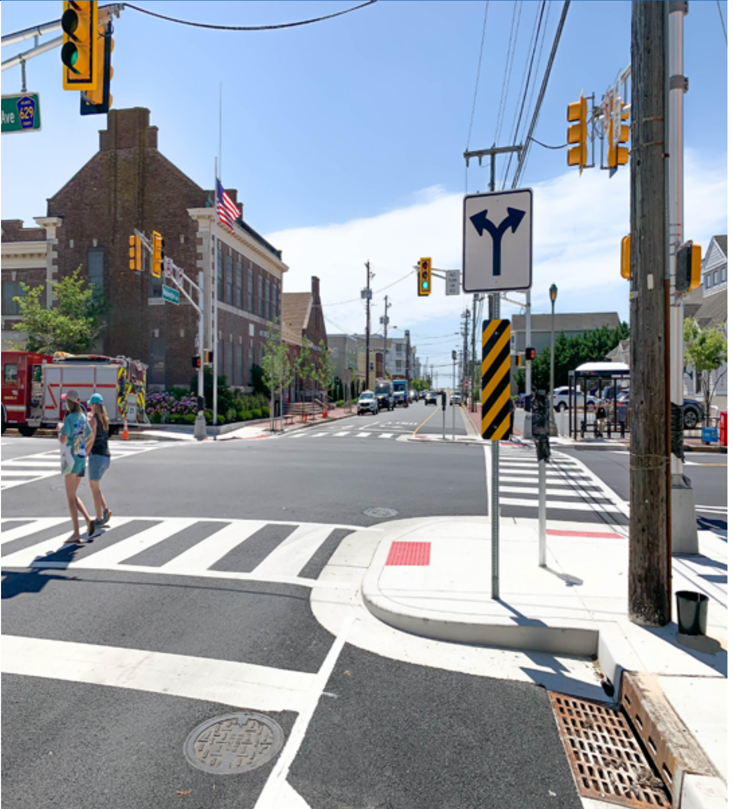
Atlantic County, Route 629 Pedestrian & Traffic Signal Improvement. SFY2021 Loan: $11,615,000
