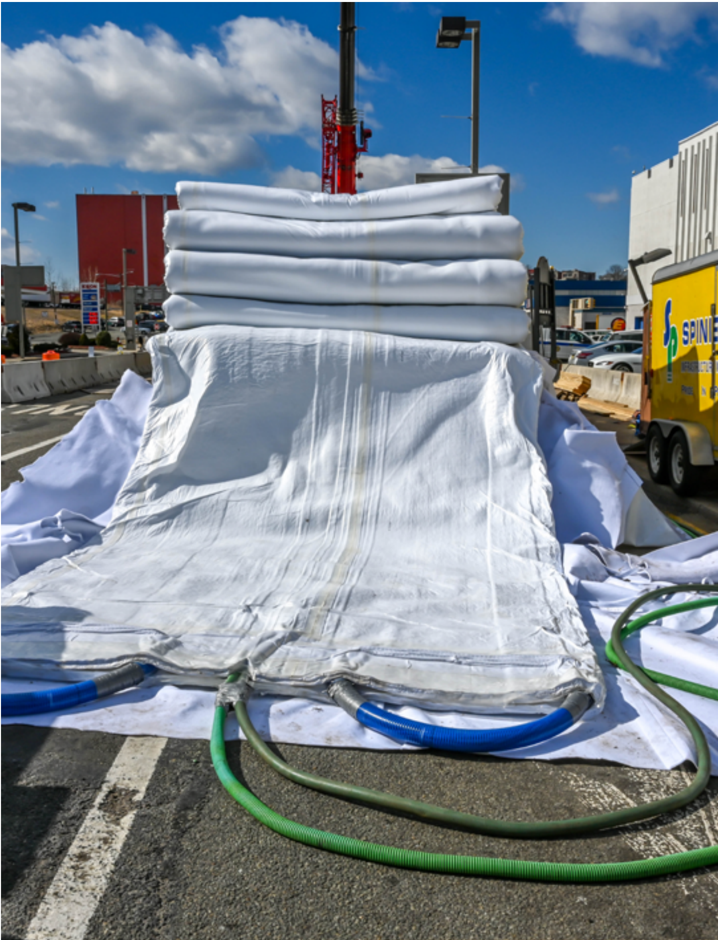
Jersey City MUA, Sewer Main Rehab. SFY2021 Loan: $1,048,438
