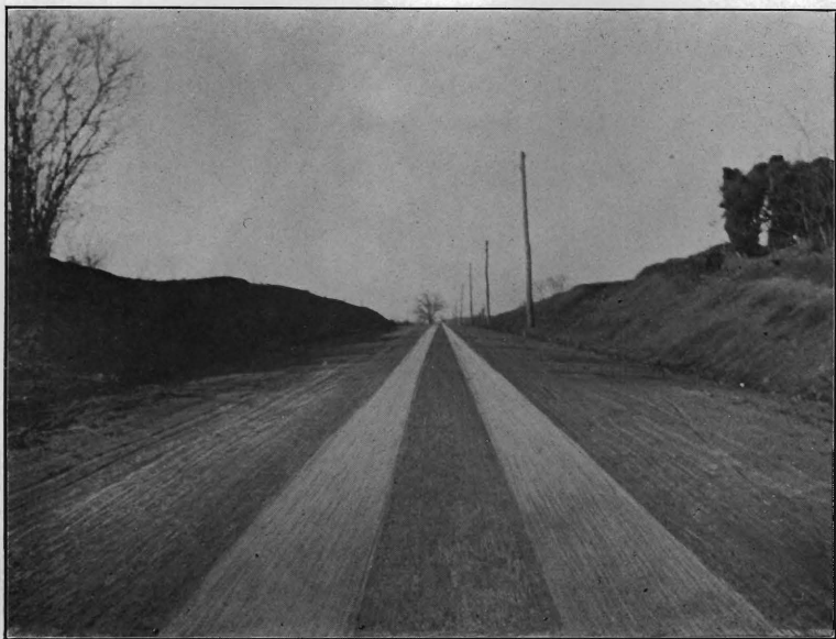
East Passaic Avenue, Essex county. 8-inch Telford pavement through deep cut.
