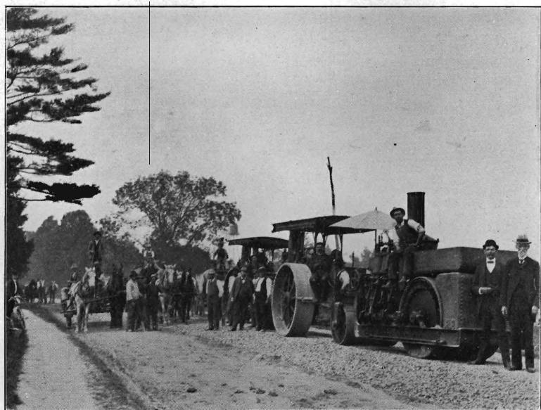
Three Steam Rollers, Water Carts and Teams At work on Old York Road, Mercer county.
