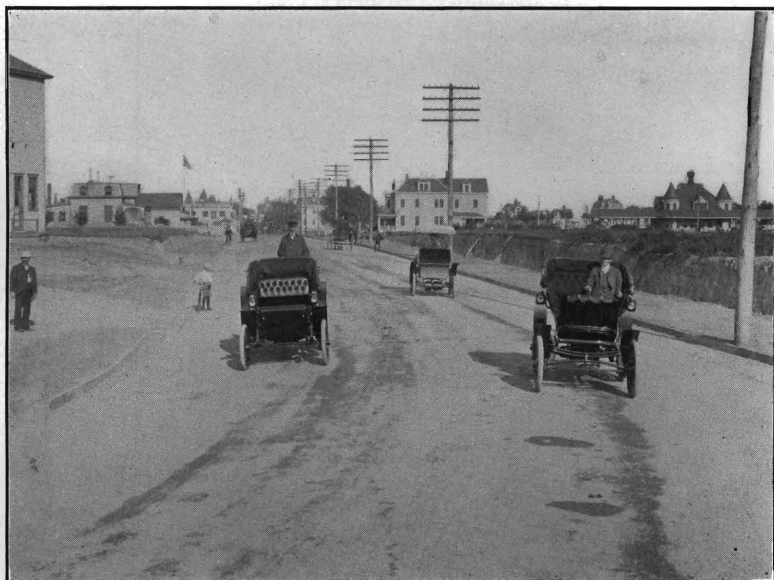
Brighton Avenue, Long Branch, Monmouth county. 8-inch macadam. 8-inch stone centre and gravel sides.
