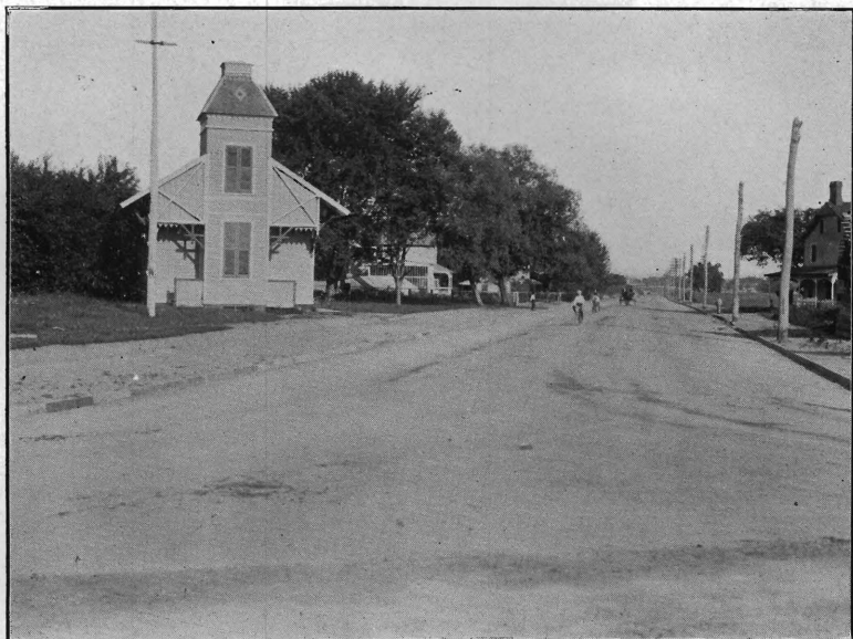
Brighton Avenue, Long Branch, Monmouth county. Finished roadway, stone centre 16 feet wide, and gravel sides. 8 inch macadam.
