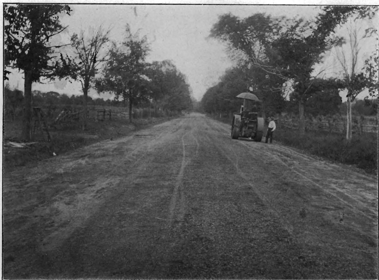
Mountain Avenue, Union county. During construction. 12 feet wide, 6 inches deep.
