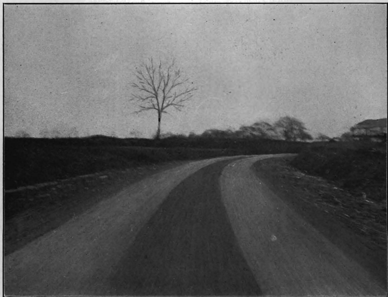
East Passaic Avenue, Essex county. 8-inch telford. After improvement. Deep cut.
