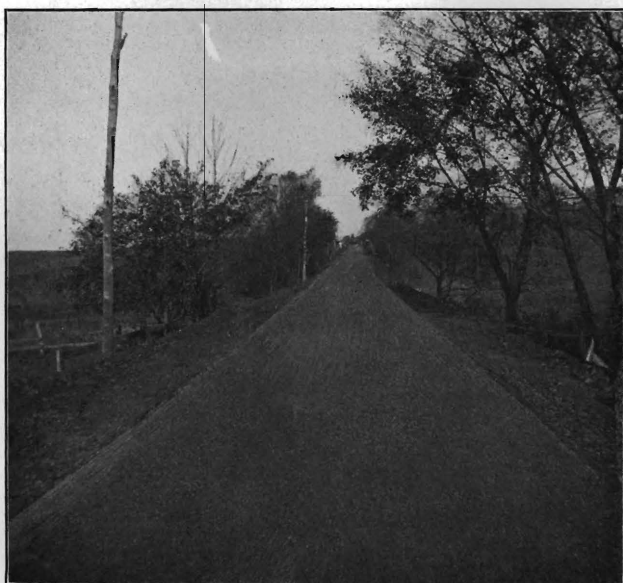
Georgetown Road, Burlington county. After improvement. 8-inch macadam, showing heavy fill.
