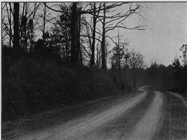
Passaic Avenue, Hudson county. After. Showing deep cutting 20 ft. wide. Telford 10-inch. Macadam, 8-inch.
