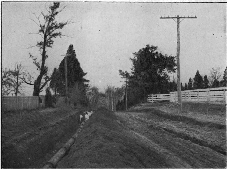
Woodbury and Knight's Run Gravel Road, Gloucester county. Before improvement. Sinking water pipe. Clark's Hill looking north.
