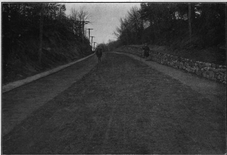
Old Bridge and New Brunswick Road, Middlesex county. After improvement. 8 inch macadam. Showing heavy cut.
