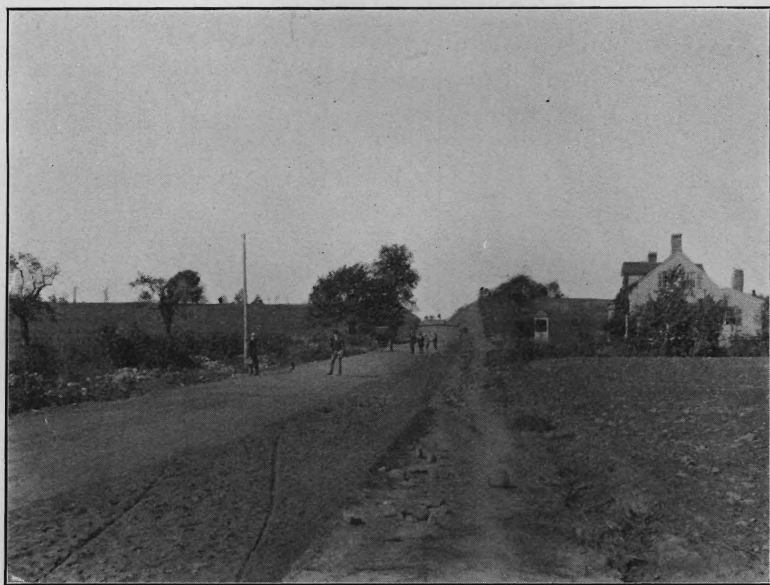
Centre Street, Franklin Township, Essex county. Showing deep cut. Telford 16 feet wide and 8 inches deep.
