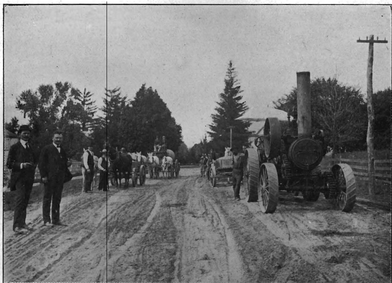
Traction Engine, Old York road, Mercer county, drawing twelve wagon loads of stone of two tons each.
