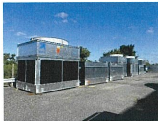
New Rooftop Equipment Delivered On-Site
