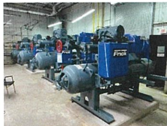
Chilling Plant – New Equipment Installed
