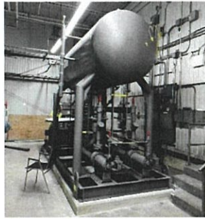
Chilling Plant – New Equipment Installed
