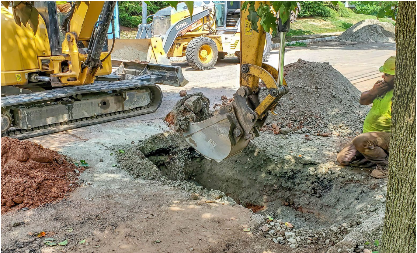
Bloomfield Township Lead Service Line Replacement. SFY2024 Financing Program.
