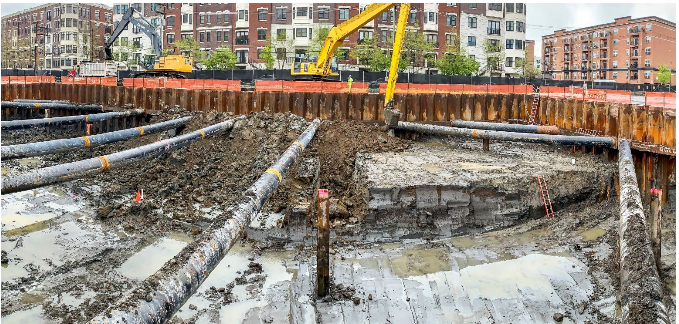
Hoboken City Southwest Resiliency Park - Acquisition, Rehabilitation. SFY2024 Financing Program.
