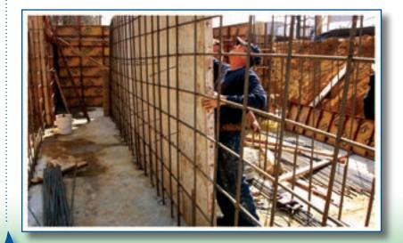
A construction worker ties steel rebar for wall reinforcement at the Millville City drinking water treatment plant.
